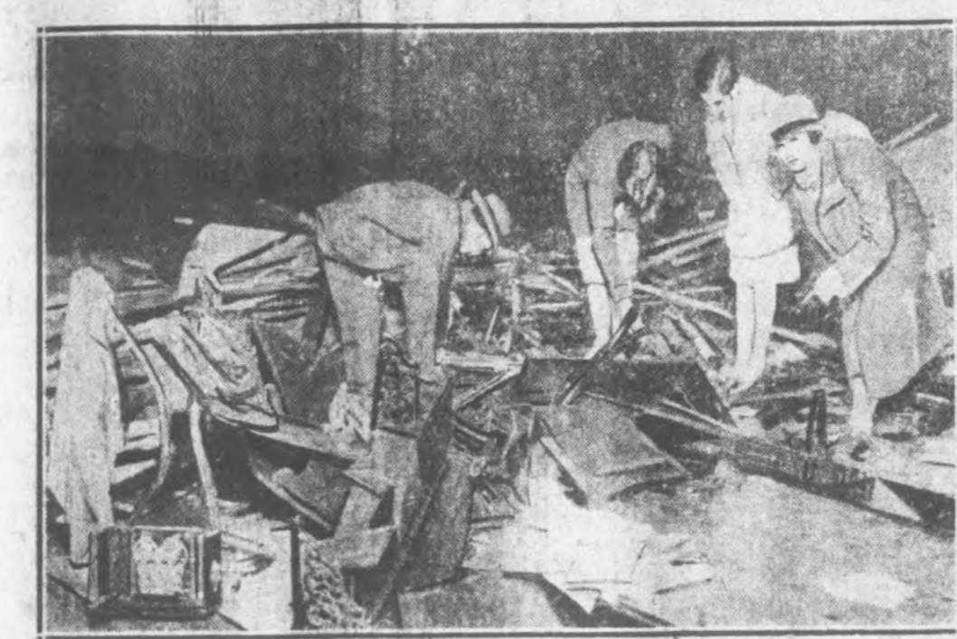
Ruins of a school at La Plata, Md., were searched after a cyclone leveled the building crushing out the lives of thirteen pupils.
