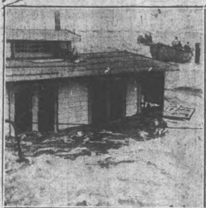
Great damage was done by storms that swept the coast of Florida. This shows wreckage at Biscayne Bay, Miami. (International News)
