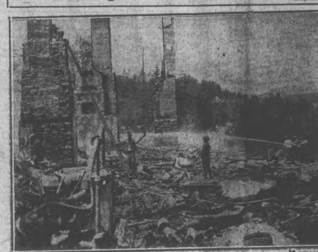
Rescue workers cooled the smoldering ruins to enable them to search for bodies of victims of the fire that destroyed Twilight Inn, Haines Falls, N. Y. Many were killed.
