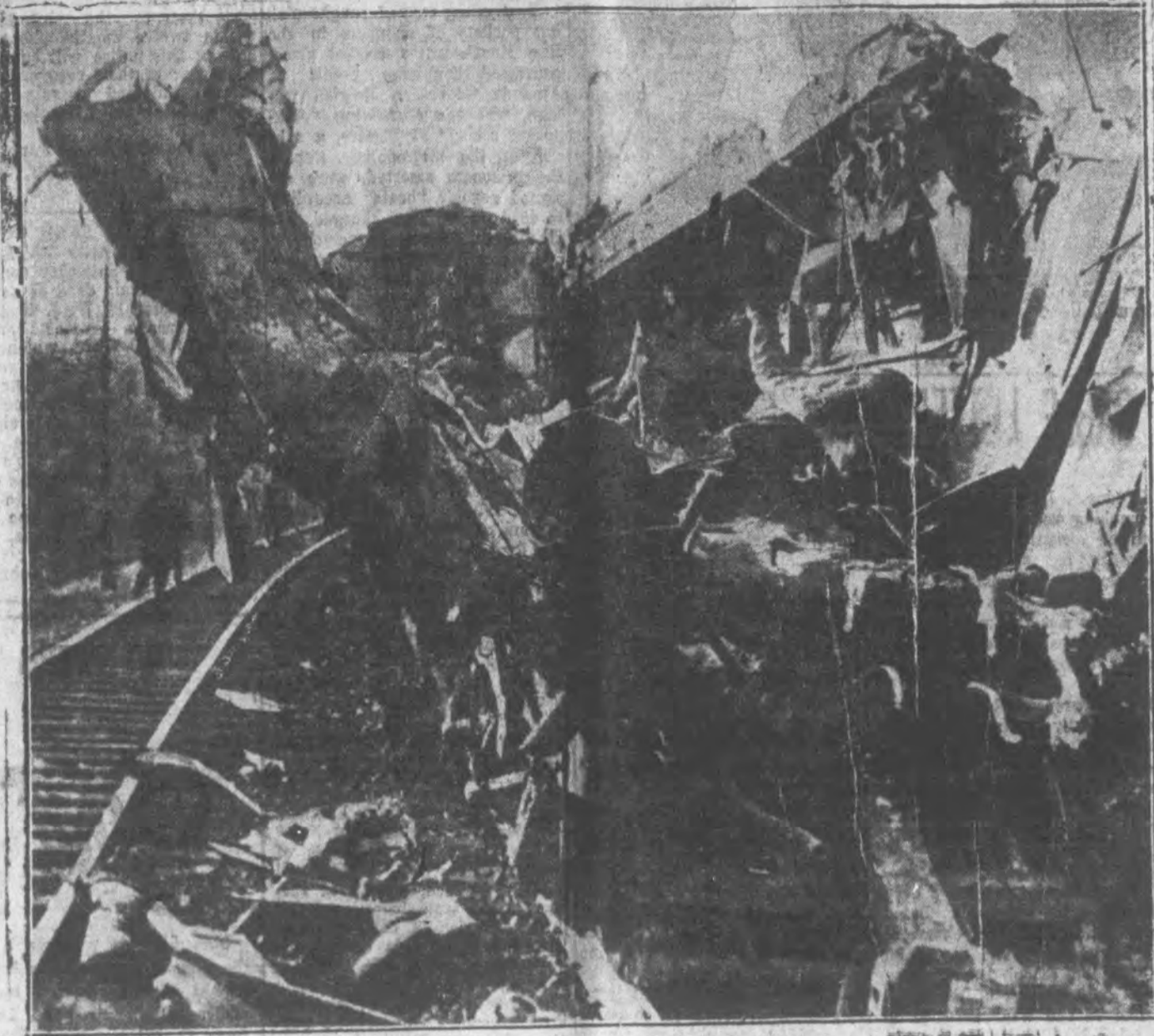
Steel splinters, and twisted iron and steel is all that remains of the wrecked portions of the two crack Pennsylvania Railroad trains which figured in a rear-end collision, near Gray, Pa. Fifteen were killed, and the number of injured was estimated as high as fifty. This picture shows the side of a steel car twisted and standing upright on the track. Many victims were removed from this pile of debris.
