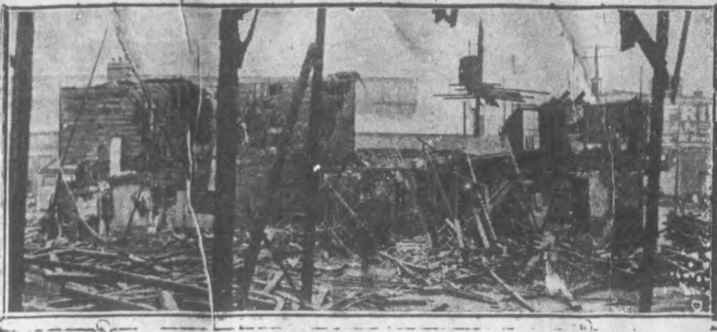
Eight persons, members of two families, were killed when fire destroyed these two homes at Canarsie, N. Y.
