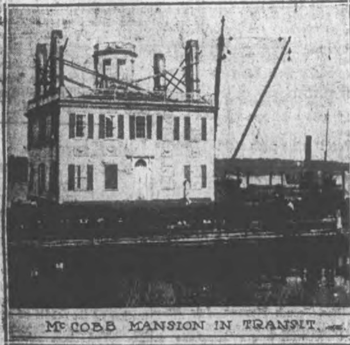
McCobb mansion in transit. The well-known McCobb mansion, built at Phippsburg, Maine, 109 years ago for Captain McCobb, was moved from there, by lighter, to Rockport, a distance of eighty-five miles, where it will be the Summer home of Donald D. Dodge, of Philadelphia.
