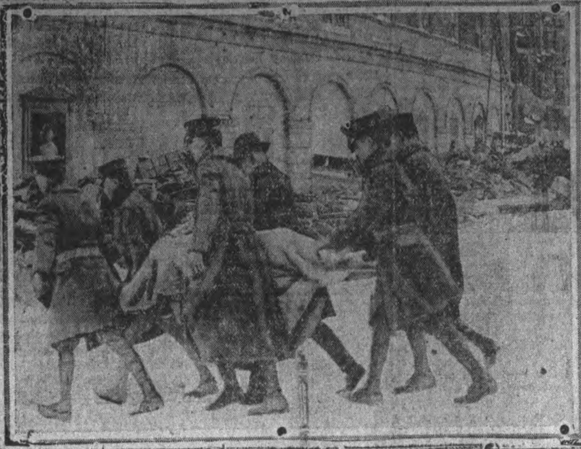
Marines carrying wounded from the ruins of the Knickerbocker theatre, Washington, D. C., which collapsed under the weight of a two-foot snow Saturday night.
