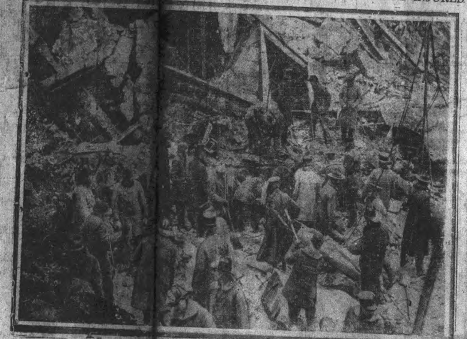
A view of the Knickerbocker theatre, Washington, D. C., showing soldiers, firemen and civilians aiding in the search through the debris for the dead and wounded. Note in the centre of the picture two stretcher-bearers carrying out a wounded person to awaiting ambulances on the outside.
