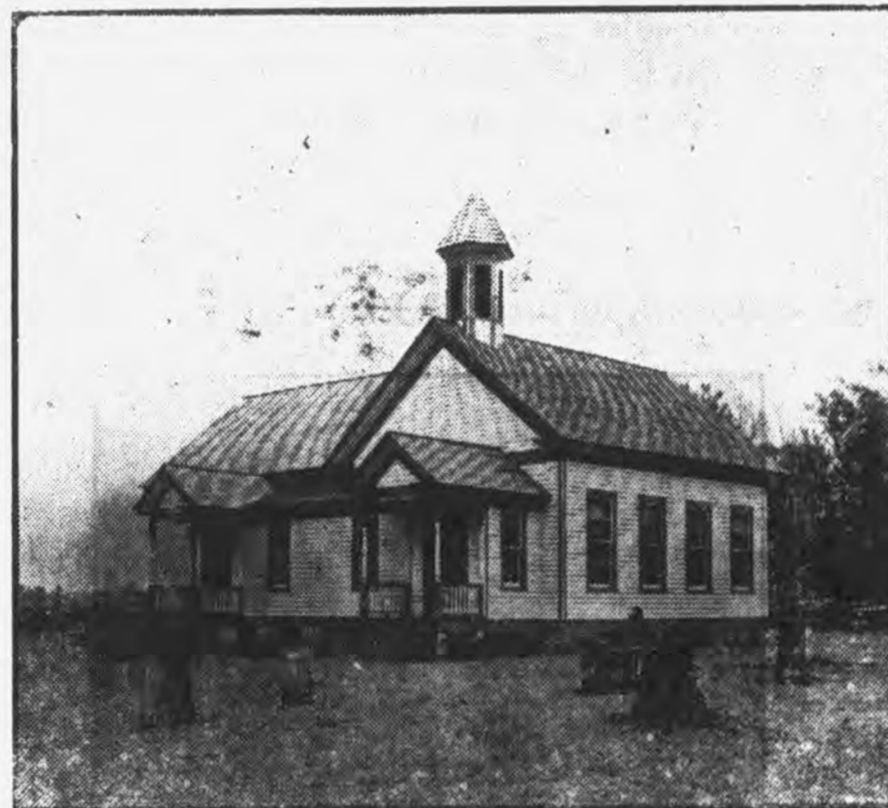
COUNTY SCHOOL BUILDING-DISTRICT NUMBER 1.
