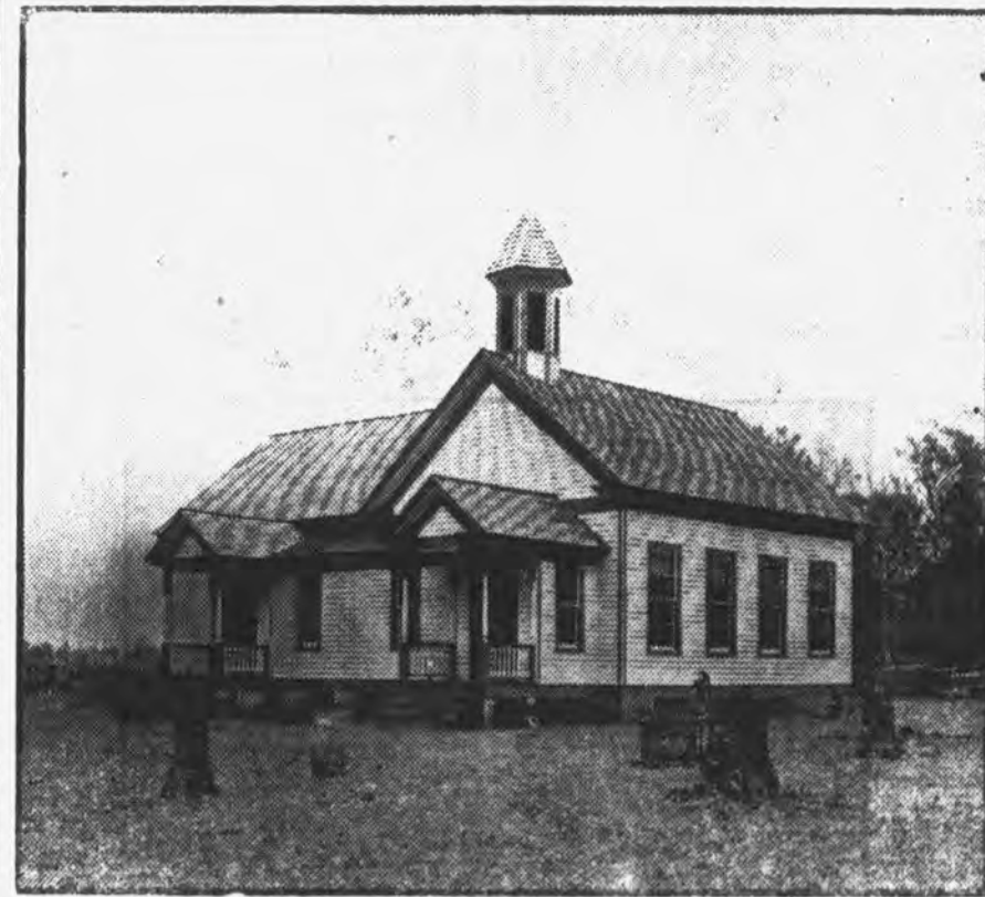
COUNTY SCHOOL BUILDING—DISTRICT NUMBER 1.
