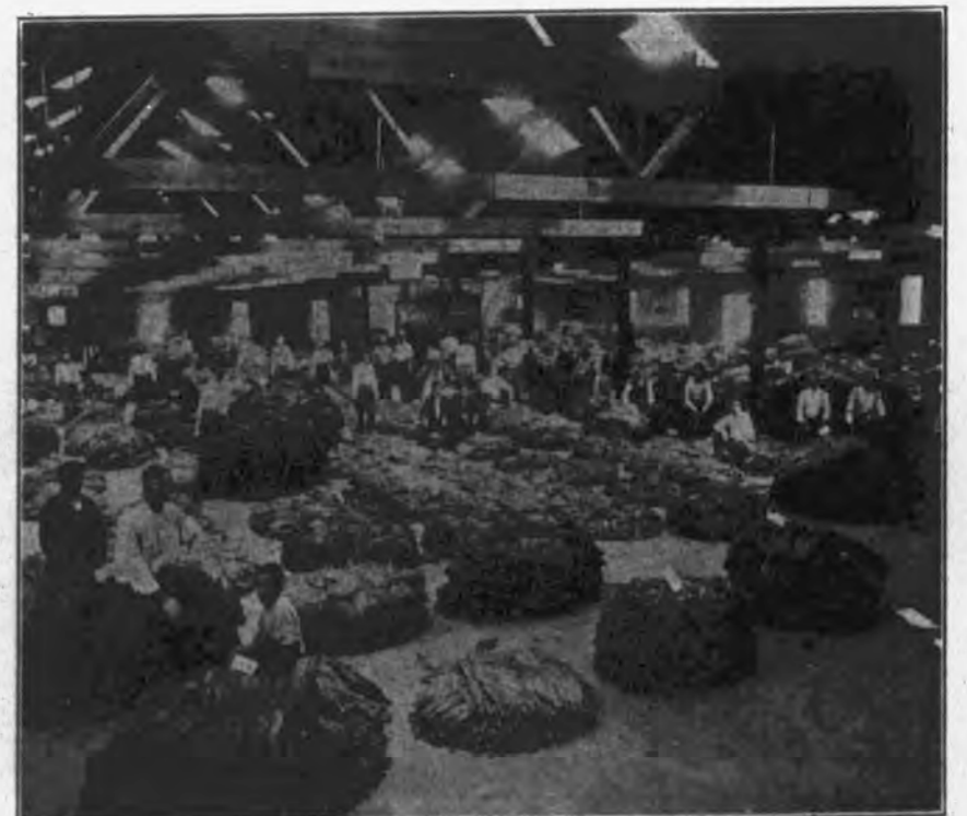
FLOOR OF CENTRE BRICK TOBACCO WAREHOUSE JUST BEFORE SALES
