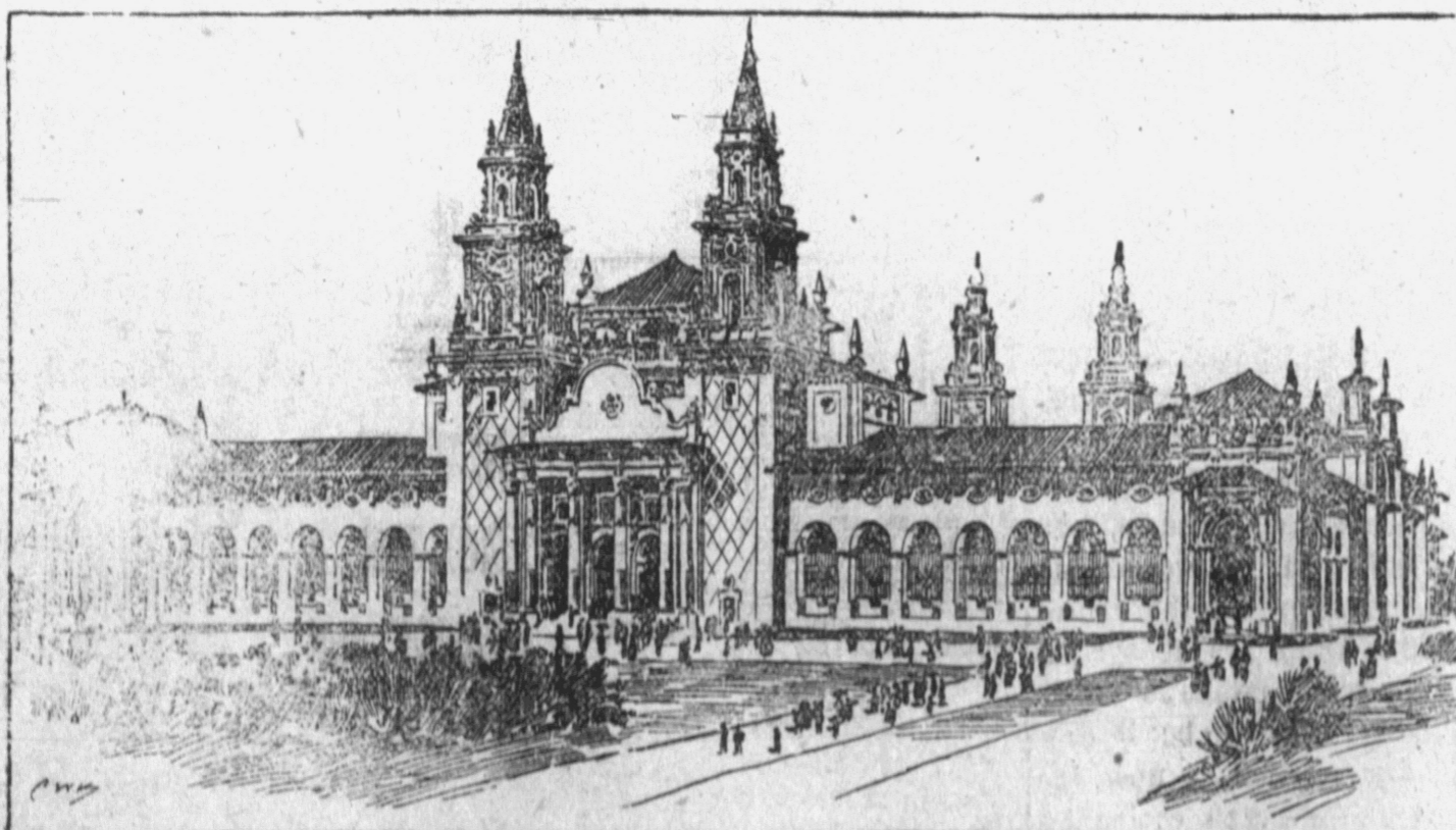
Copyright, 1900, by the Pan-American Exposition Co. This large structure is 500 by 350 feet, with a central court 100 by 175 feet. Its type of architecture is the Spanish Renaissance, modified to suit the conditions of the Exposition. The roofs are laid with red tile and the cemented walls are brilliant with color. The colors are to be reds and yellows in light tints. The facades will present an arched effect, with broad, overhanging eaves, in imitation of the old mission buildings in California and Mexico. The Central Court will be a veritable tropical garden, with a long, narrow pool, containing interesting specimens of aquatic life, and will have seats, where the weary visitor may rest a moment. The Exposition is to be held in Buffalo in 1901 from May 1 to Nov. 1.
