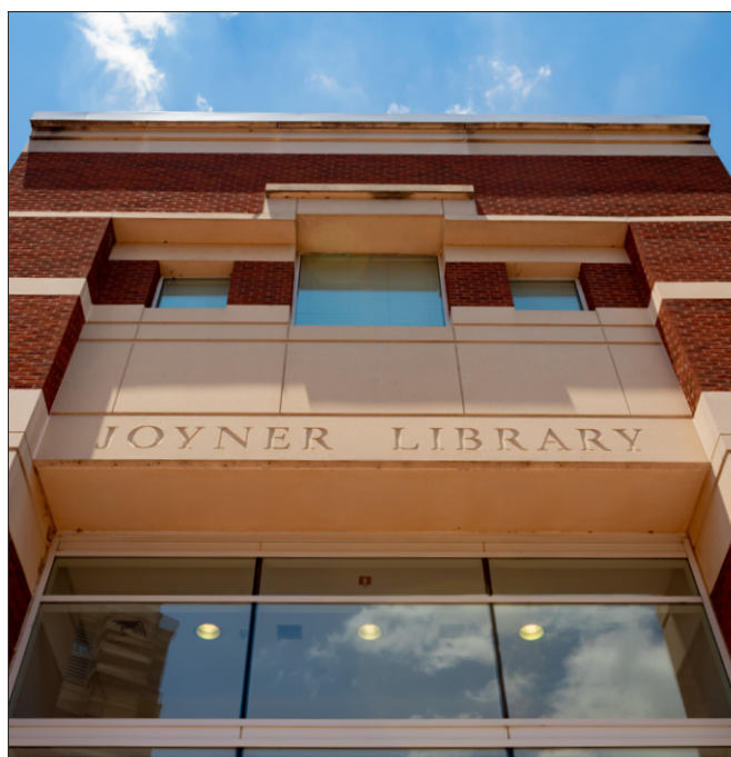
Joyner Library at ECU is one building expected to undergo review.
