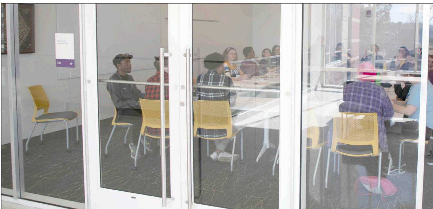
Looking through the windows outside the Dr. Jesse R. Peel LGBTQ Center, which will need to be replaced after the wrong-sized ones were installed.
