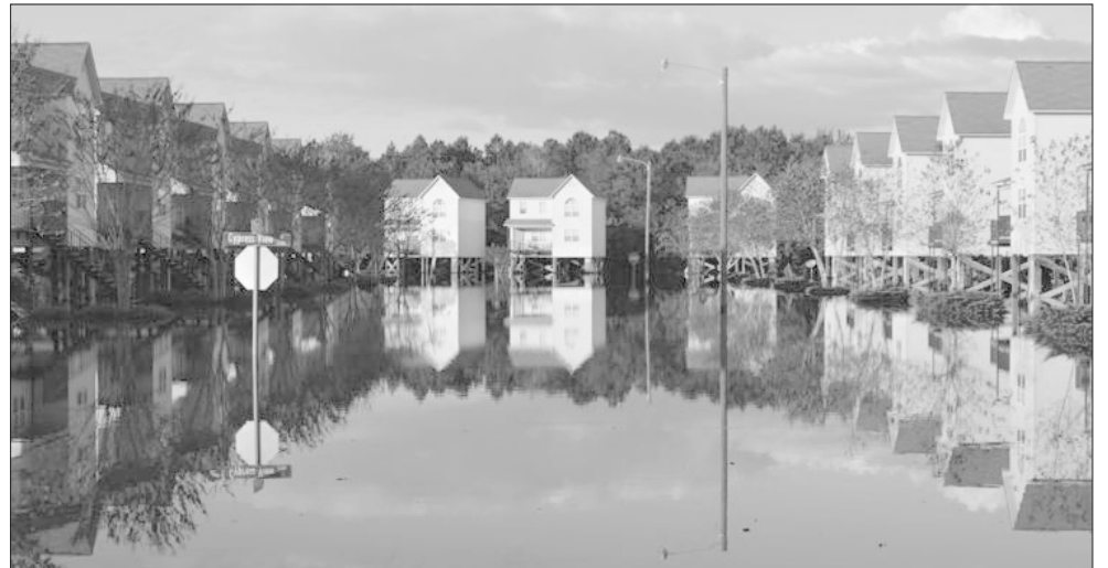
The Riverwalk Apartments experienced significant flooding after Hurricane Matthew in 2016.
