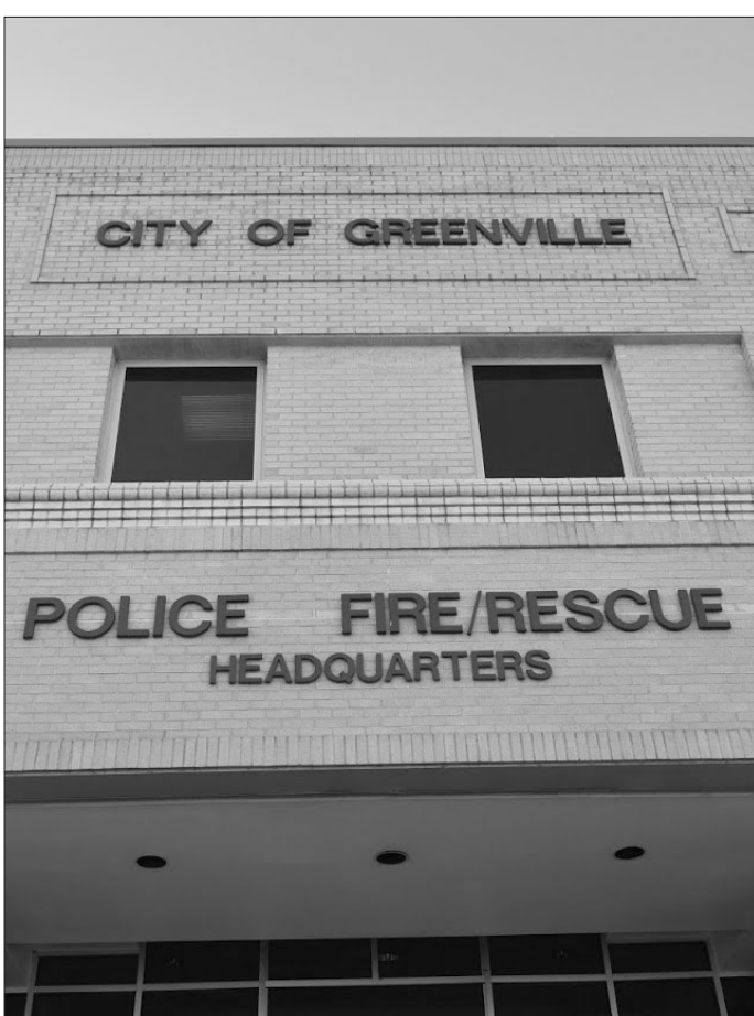
Greenville Fire/Rescue's headquarters in downtown Greenville.
