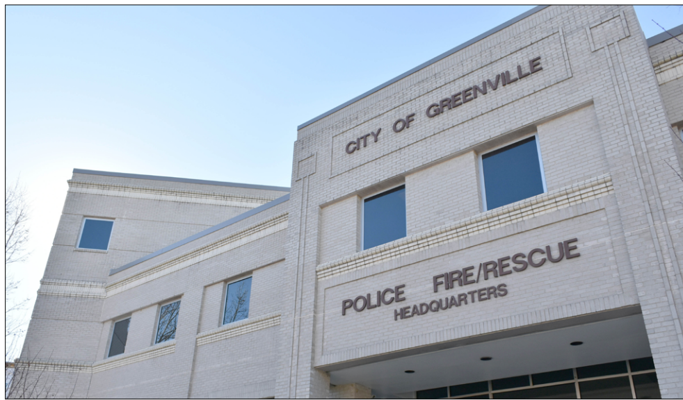
Greenville Fire/Rescue's headquarters in downtown Greenville. GFR is currently under investigation.
