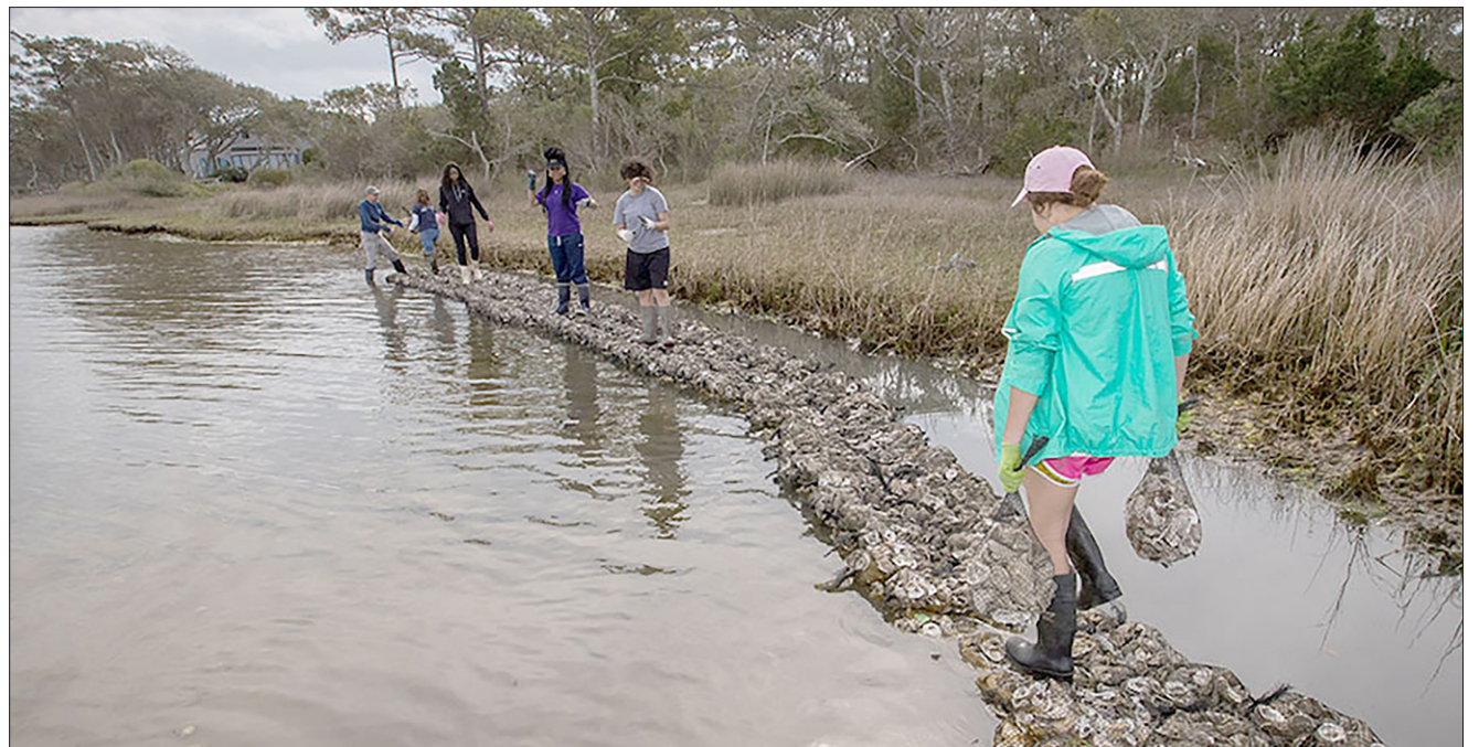
East Carolina University students help to build a living shoreline at Trinity Center at Pine Knoll Shores during spring break of 2017.
