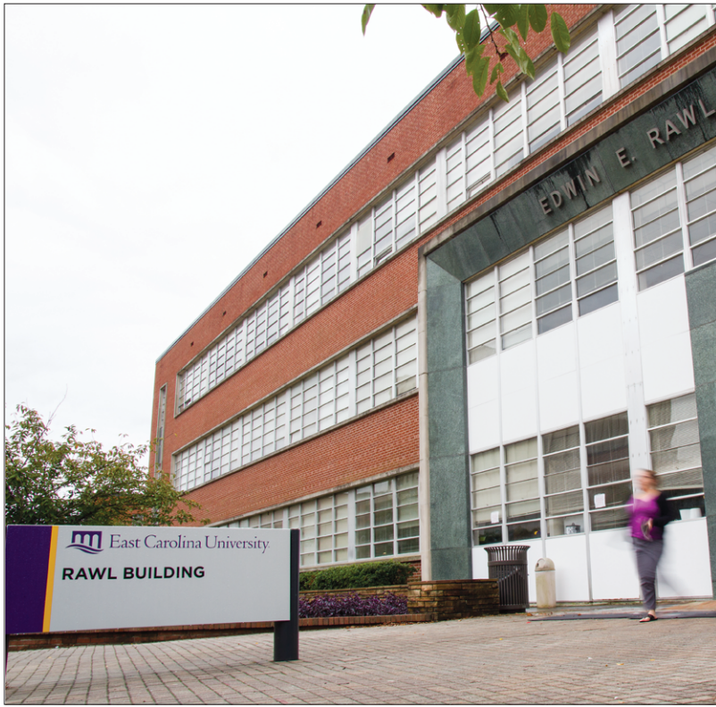
Asbestos was removed over fall break from the hallway ceilings inside of Rawl. MICHAEL SEEGARS | THE EAST CAROLINIAN
