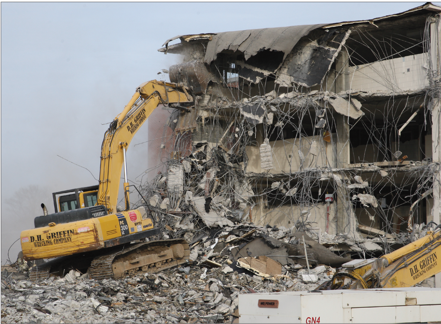
Demolition crews work on Sunday afternoon to take down parts of Belk Hall. The dorm is being torn down to be replaced by a new facility for students.
