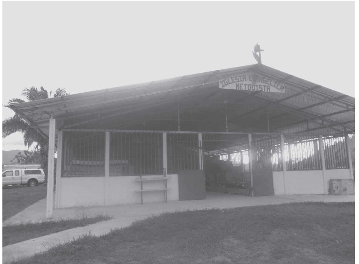
Thirteen students spent their spring break in Costa Rica building a house and a church for a preacher in need.
