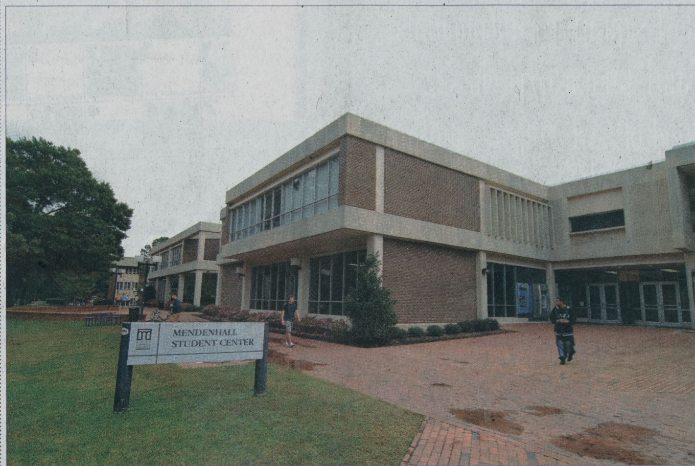
Mendenhall Student Center will continue operation for the Fall 2008 semester, pending decision about future construction.
