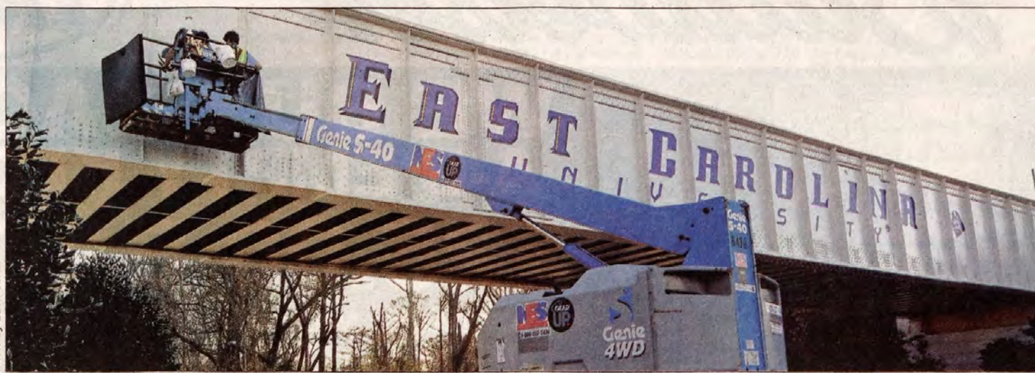
Saffo Contractors' crew works on painting Pirate logos and the words "East Carolina University" on the trestle over Charles Boulevard.
