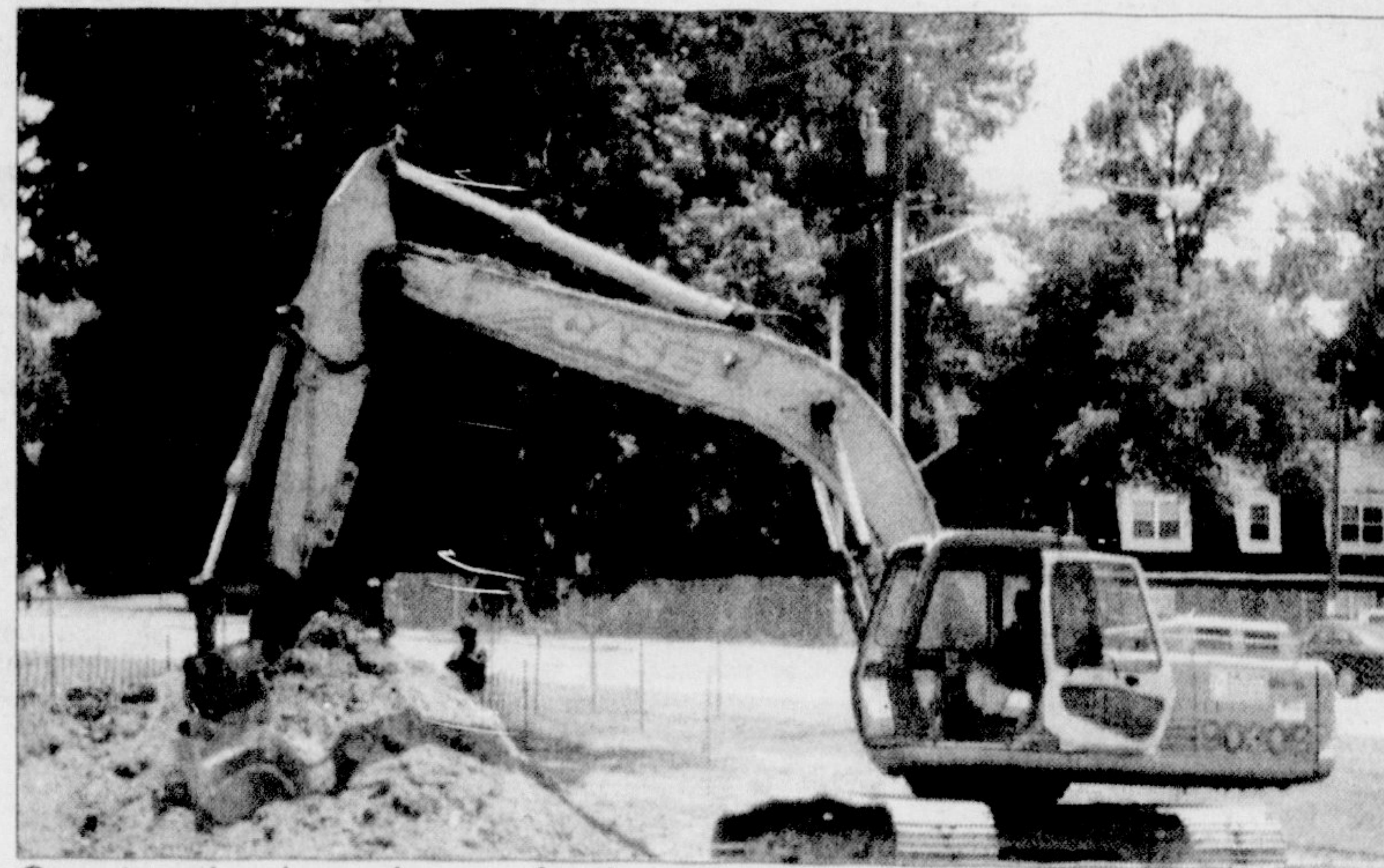
Construction is underway for the expansion of Harrington Field.
