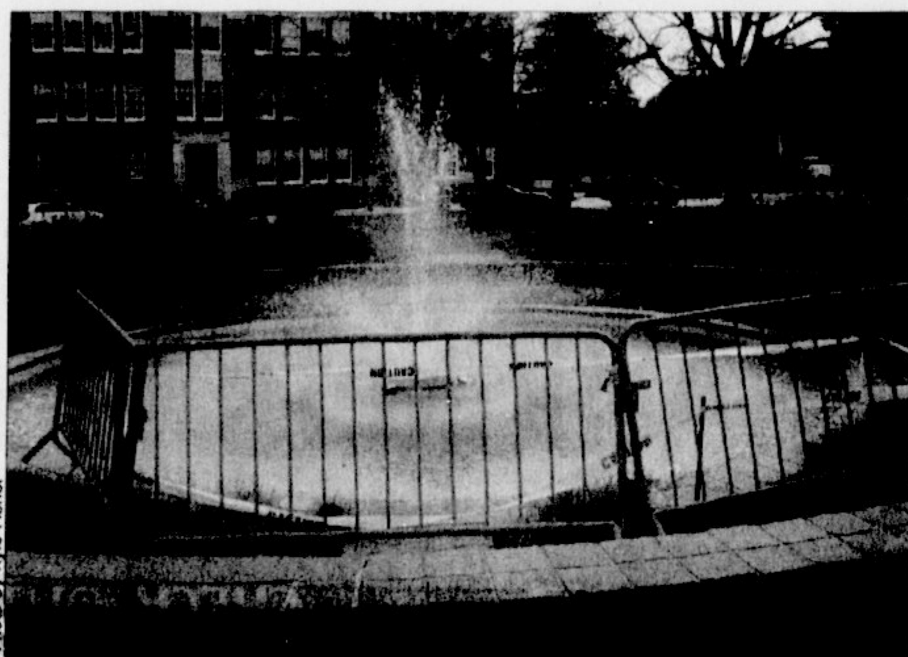
Cameras were placed under Wright Fountain to find a leak.
