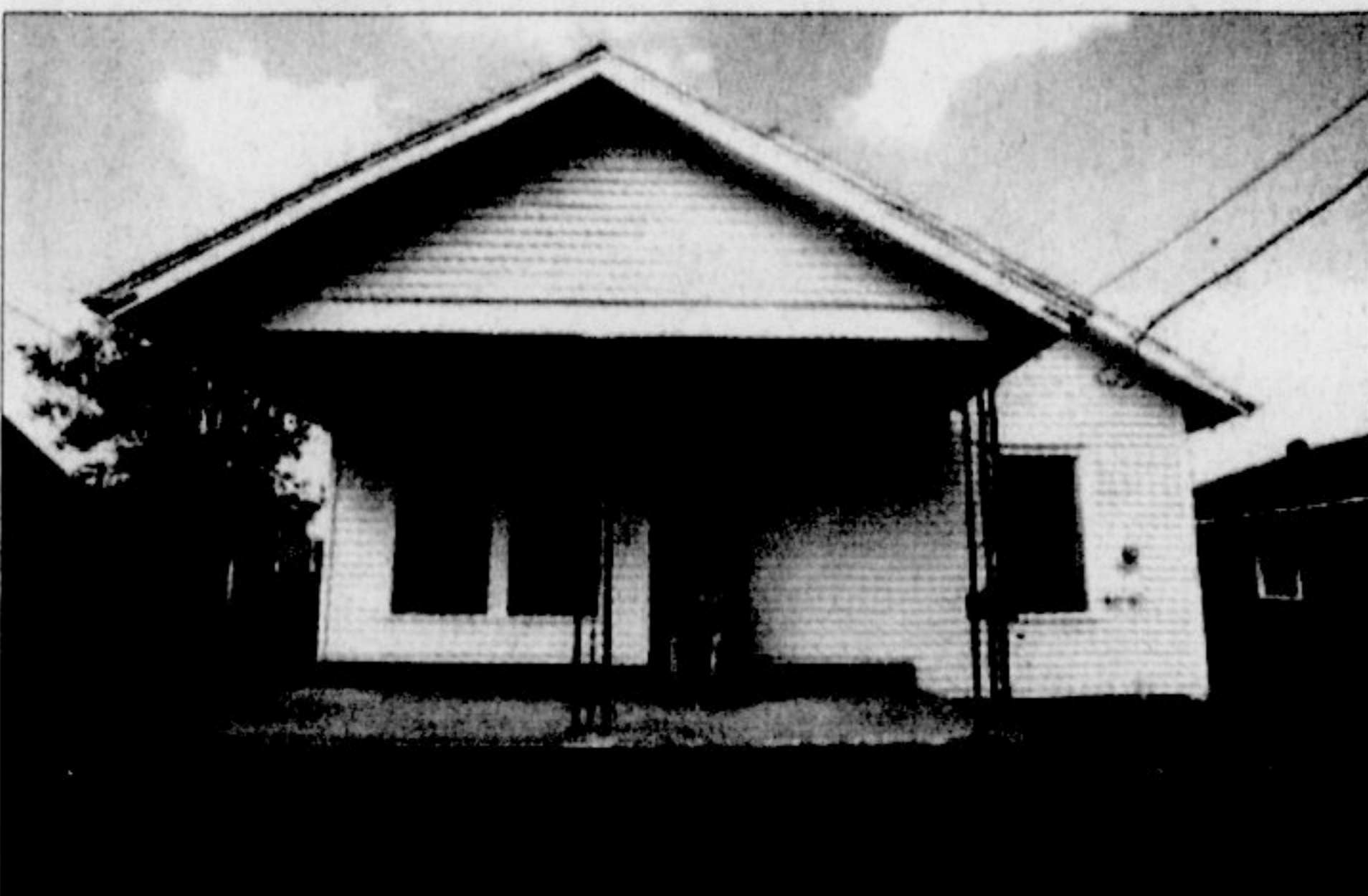
Louisiana residents deal with even more flooding after Rita.
