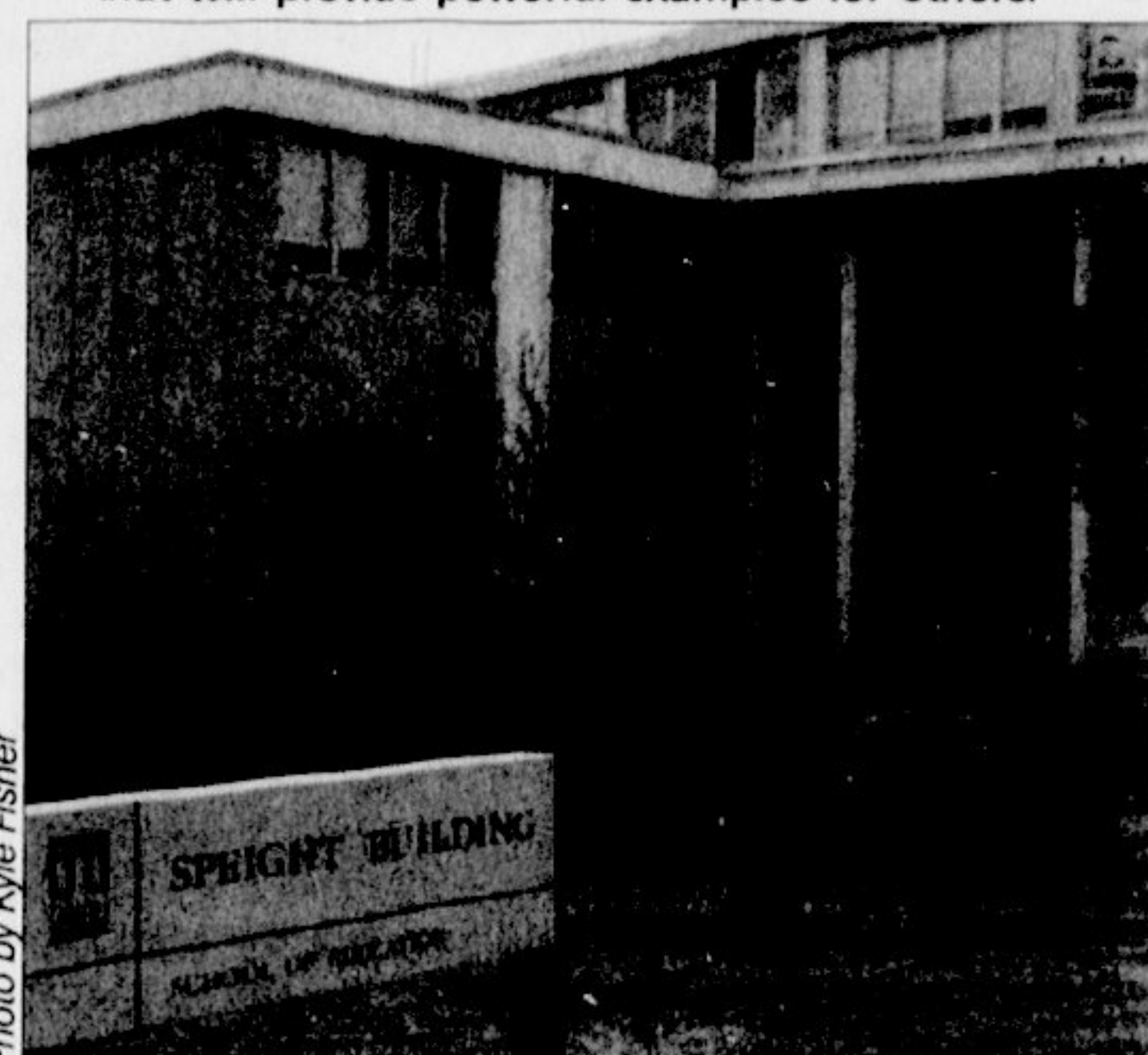
THE SPEIGHT BUILDING
