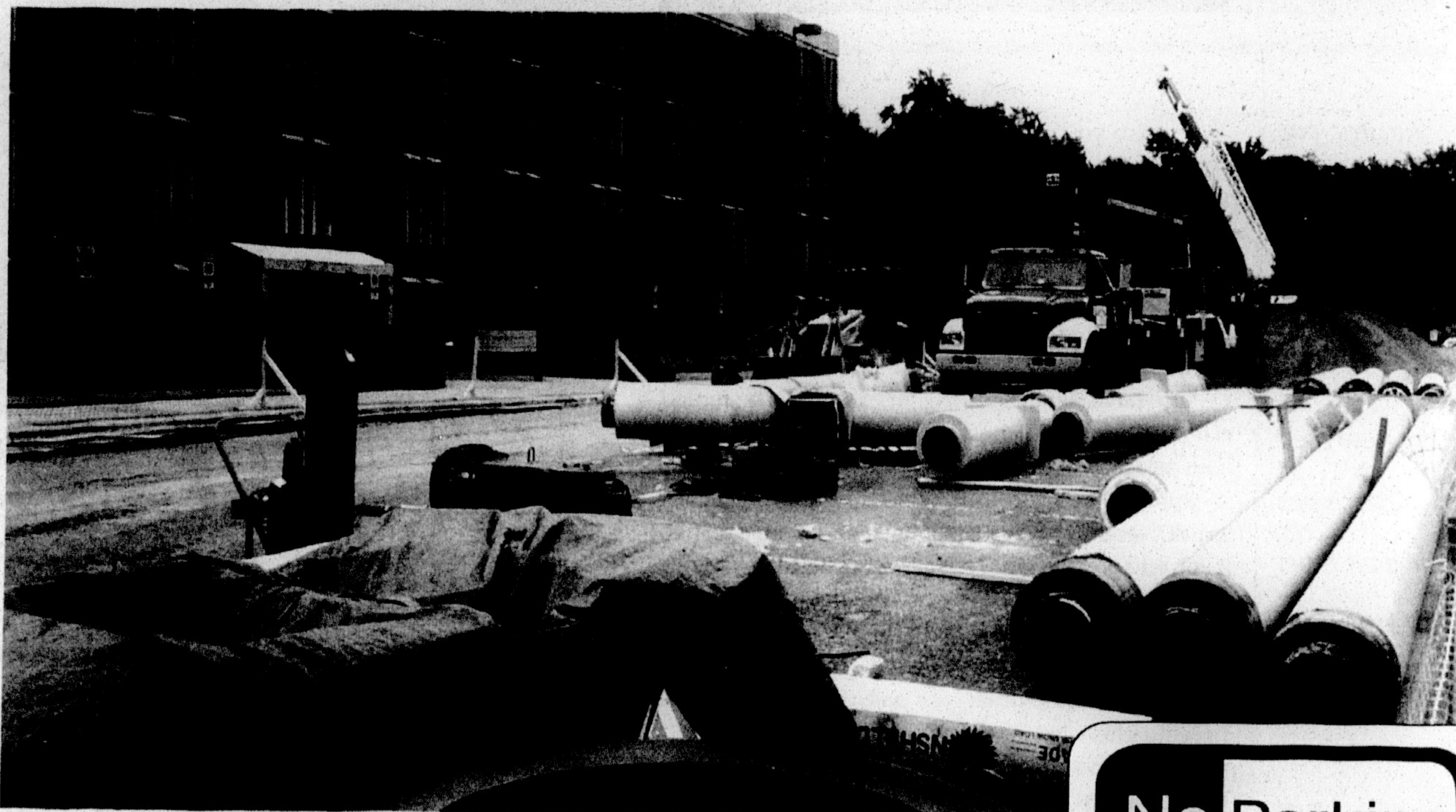
The lot in front of Christenbury has been temporarily stripped to make way for a new steamline. (photos by Shane Cranford)
