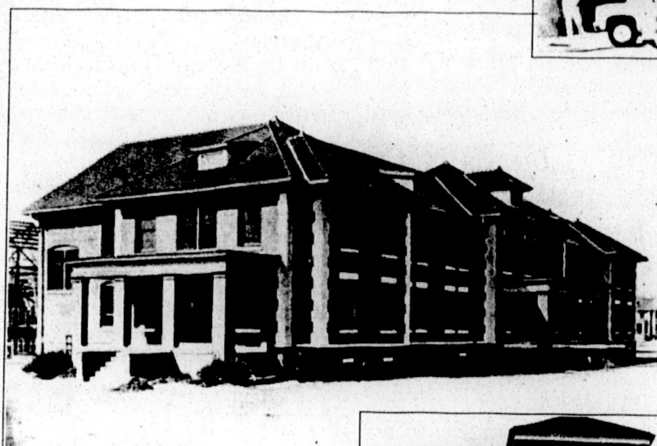
Above: Jarvis in its mid-constructed state. (photo by Garrett McMillan)
