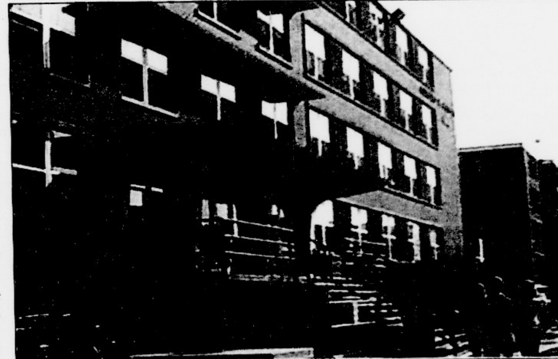
Aycock Hall, which is on College Hill Drive, was temporarily evacuated due to a fire on the third floor as students arrived back from Fall Break Tuesday night.
