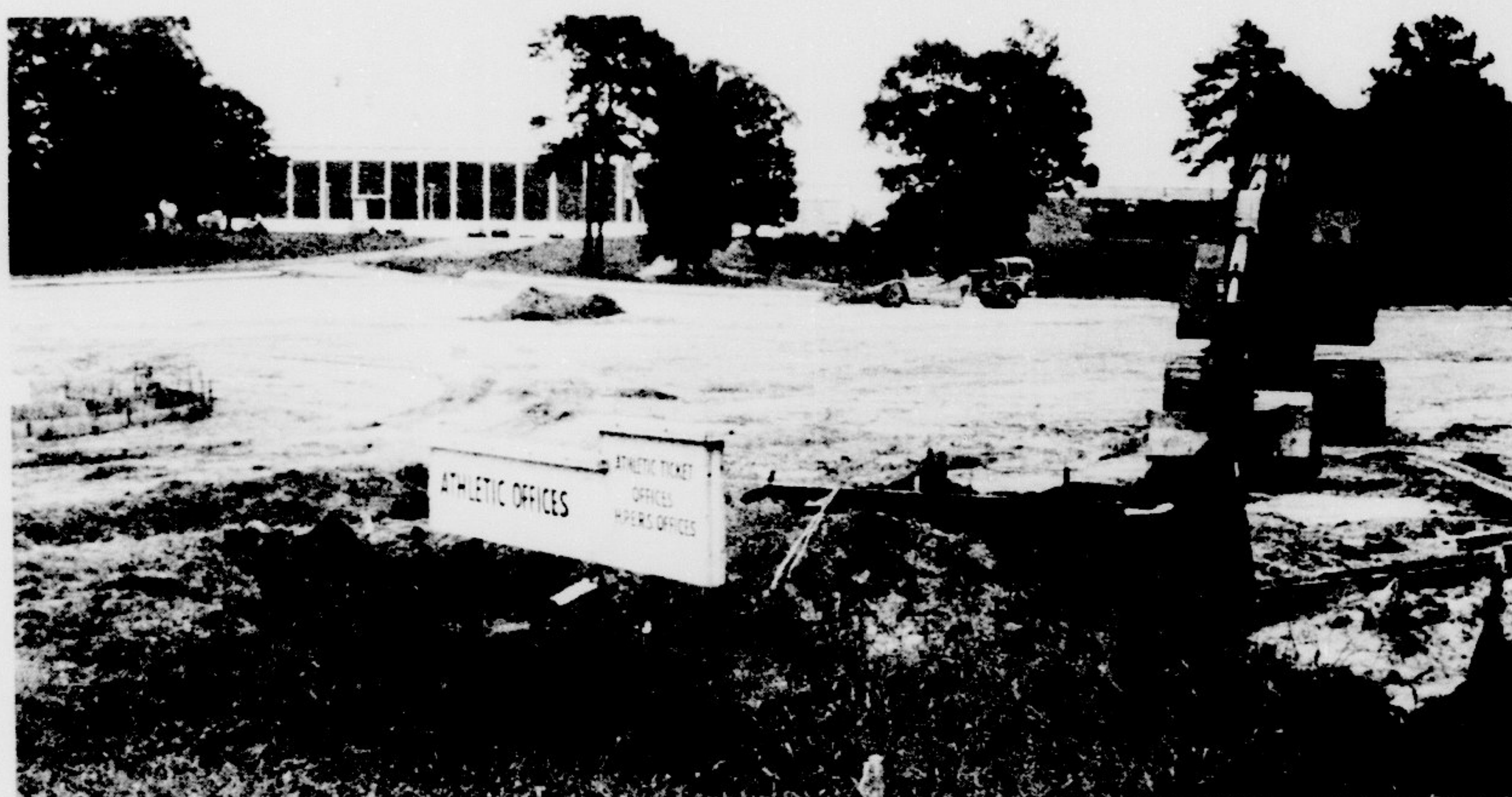
The parking lot being constructed near Minges on Charles Street will hold 586 cars when completed. (Photo by J.D. Whitmire—Photolab)
