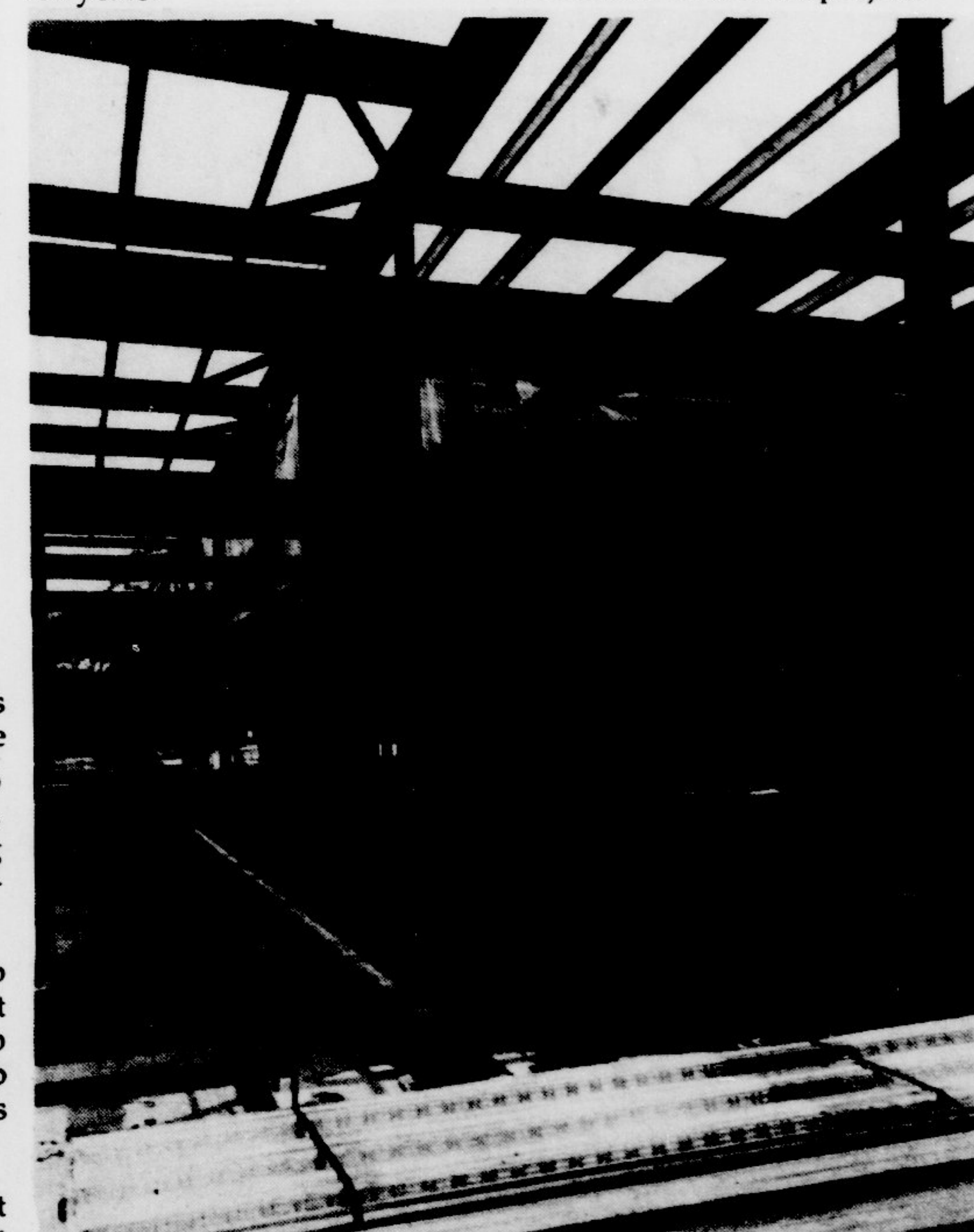
This is the skeleton of the new wing of Mendenhall Student Center which will create 31,000 square feet of new area. (Jon Jordan—Photolab)
