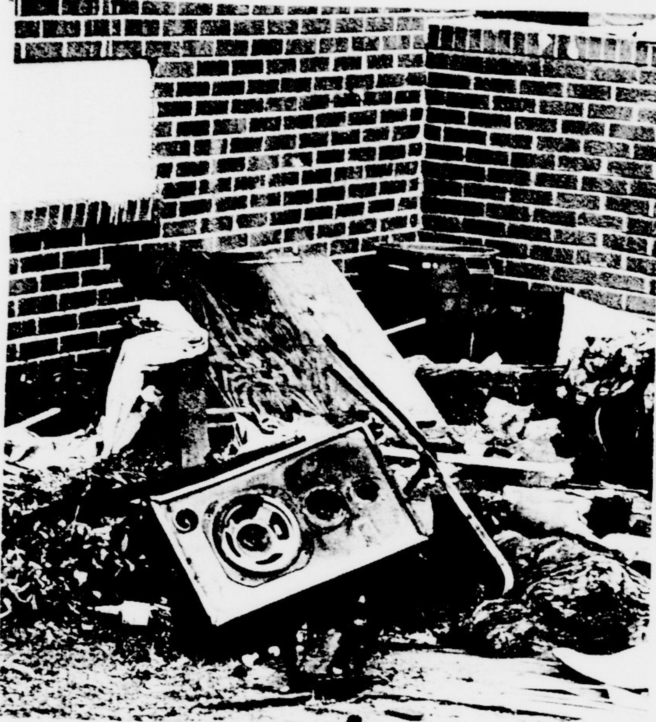
Fire caused major damage at the Tau Kappa Epsilon fraternity house Saturday morning, leaving little more than burnt rubble in many areas of the house. The structure had to be condemned because of the damage.
