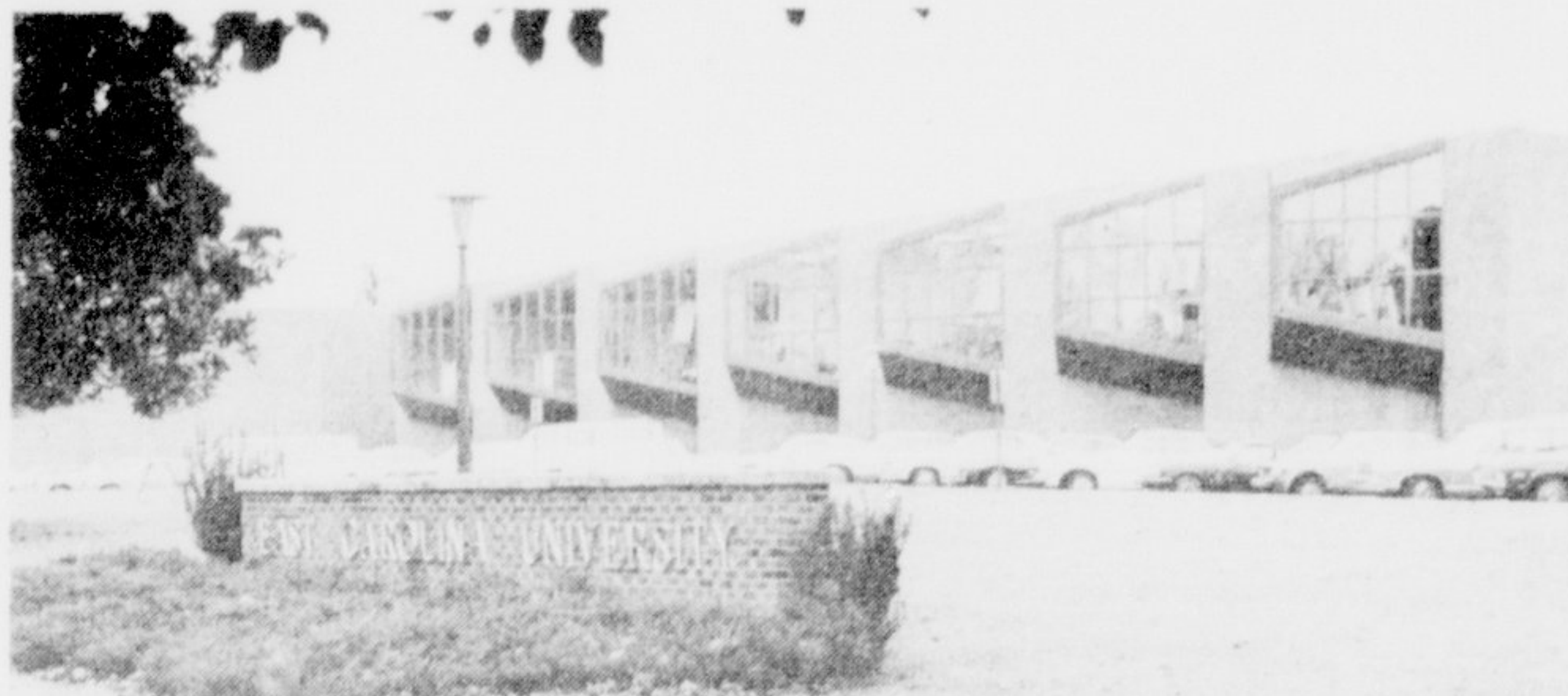
NEW ECU ART BUILDING.
