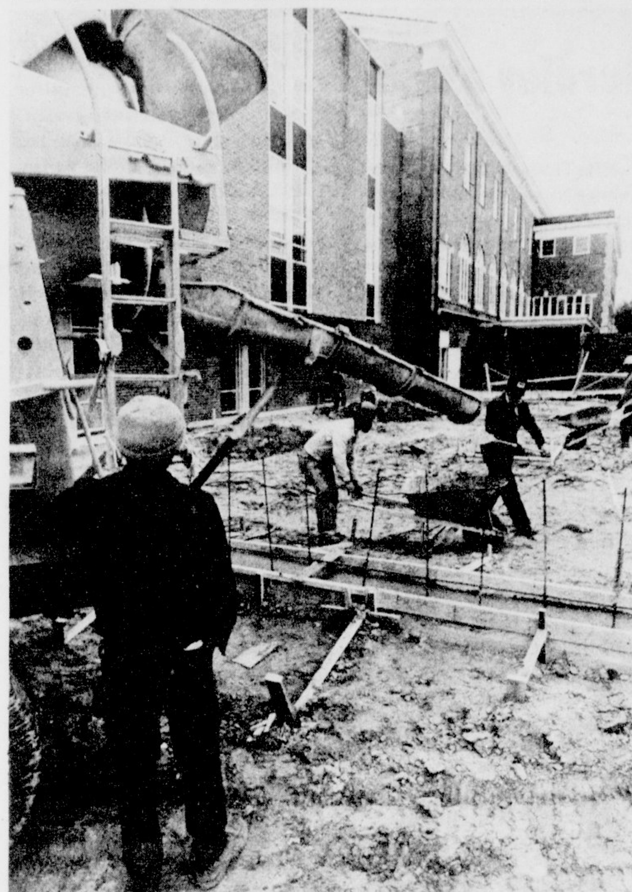
NEW WAREHOUSE site outside Wright Annex. [Photo by Brian Stotler.]
