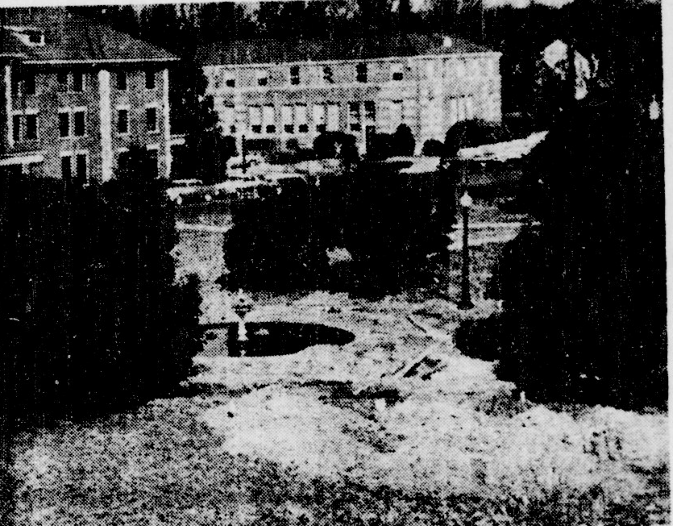
BEFORE . . . Wright Circle patiently awaits workers to begin extensive revisions.
