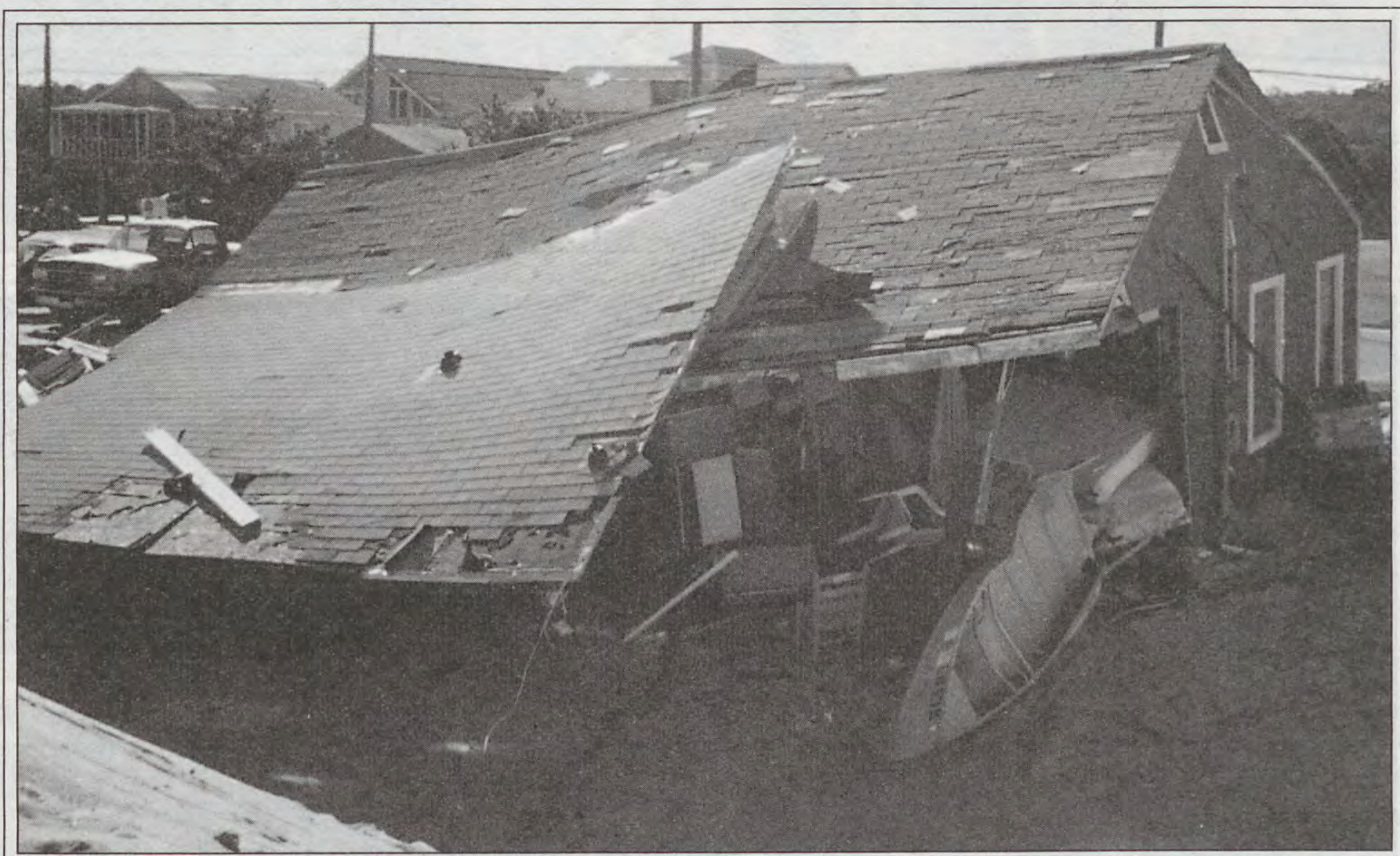
These photos (above and next page) of property in Kure Beach, NC, illustrate the damage a hurricane's wind and water can do. Photos courtesy Elizabeth W. Sapp.
