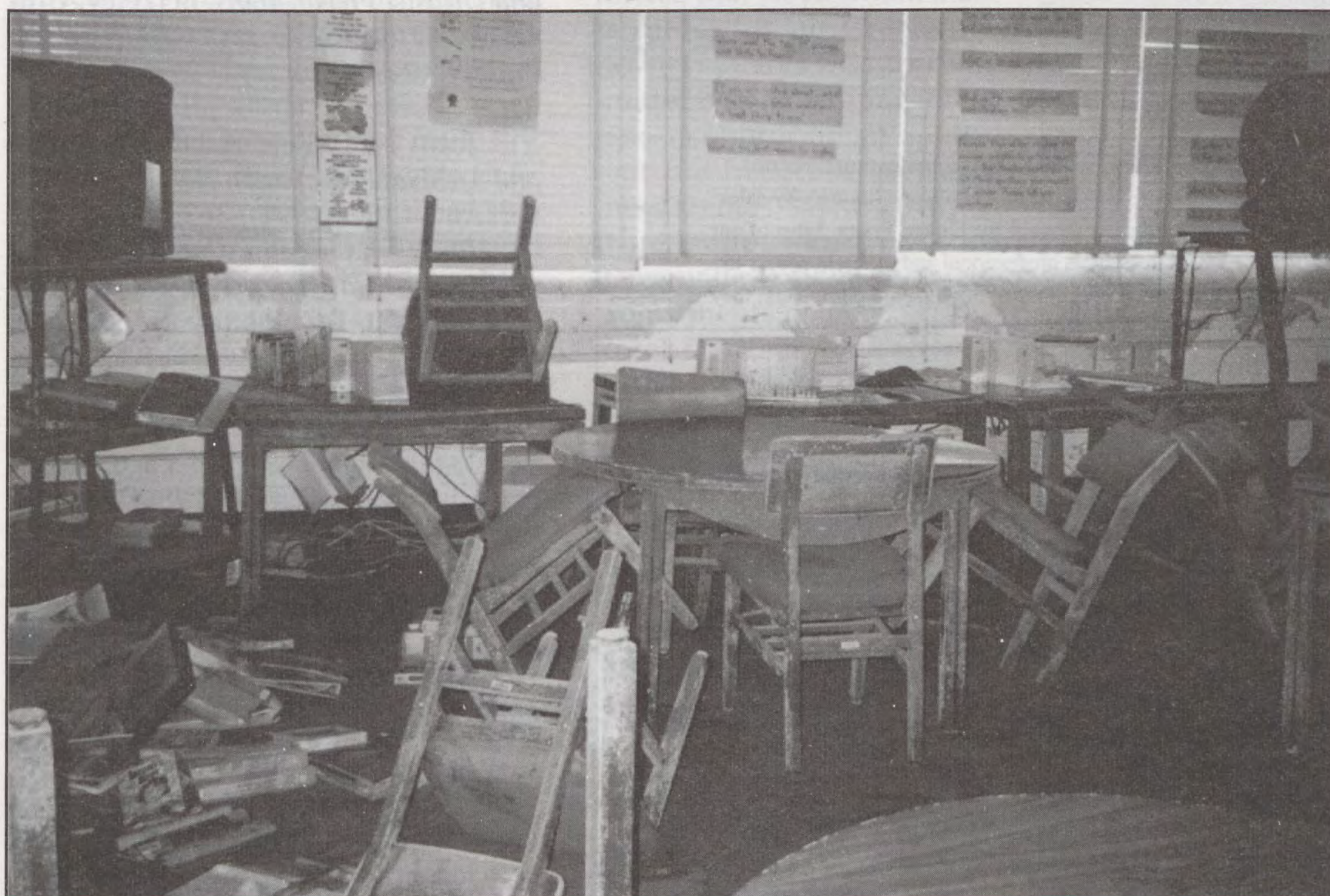
Damage to the Pattillo Elementary School library was extensive. Note the height of the water line (top photo). Photos courtesy Angie Egerton.
