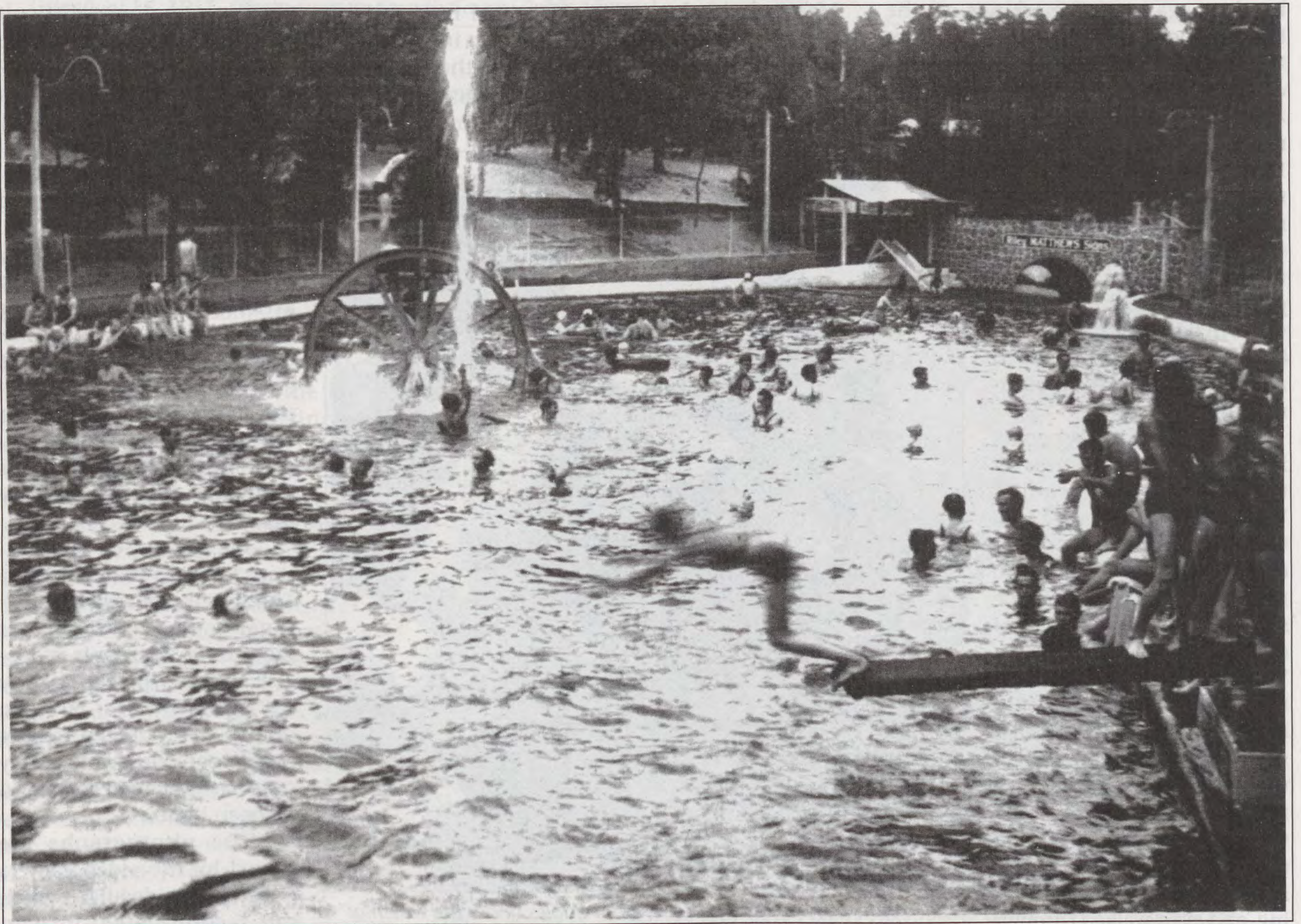
Crystal Lake swimming pool with diving boards, water wheel and fountains. The pool opened in the 1930s.
