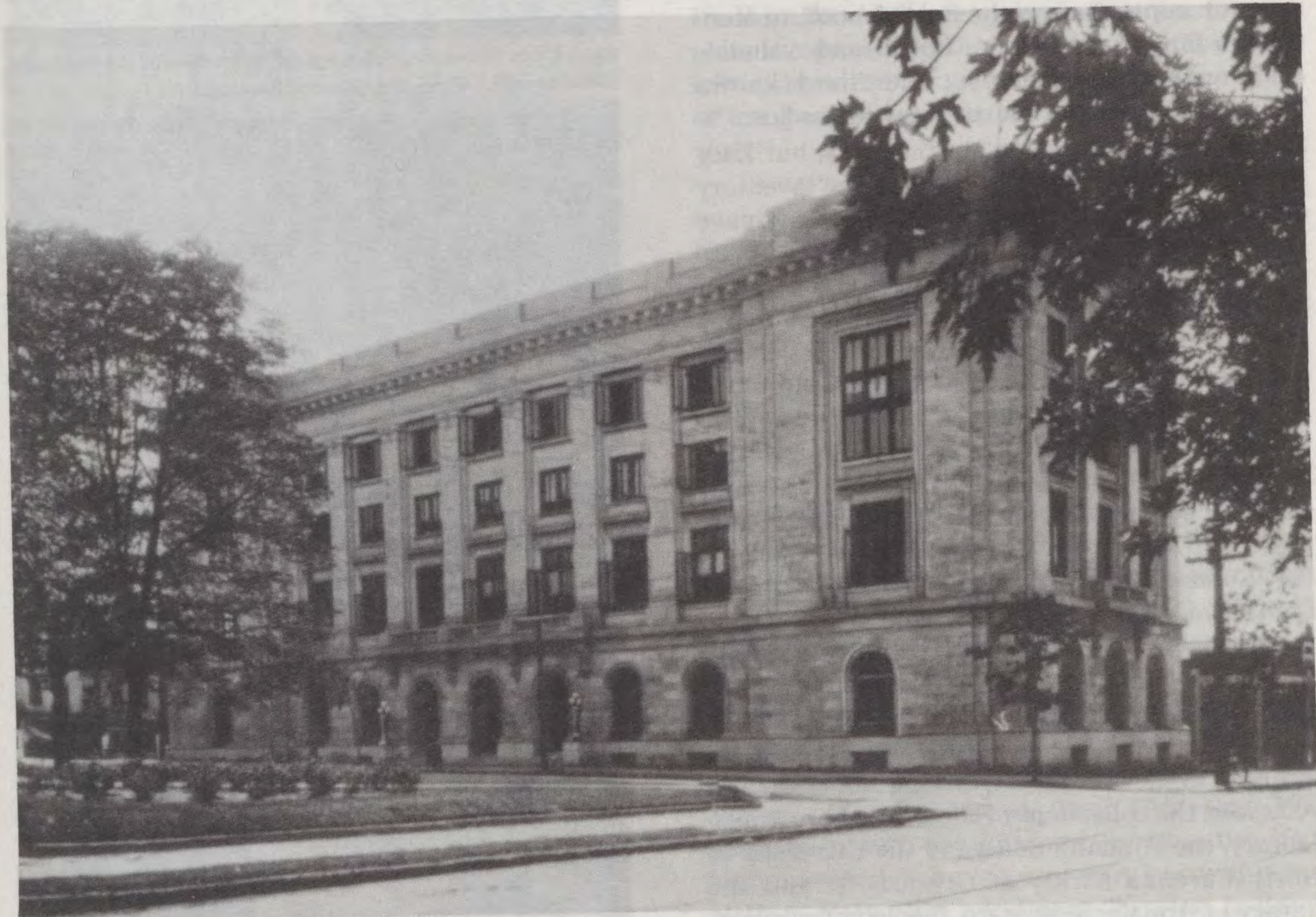
State Administration Building, located south of Capitol Square in Raleigh. The State Library occupied the first floor, and the Historical Commission utilized the second floor. The third floor housed the Supreme Court. (Photograph [circa 1914] from files of the Archives, Division of Archives and History, Raleigh.)
