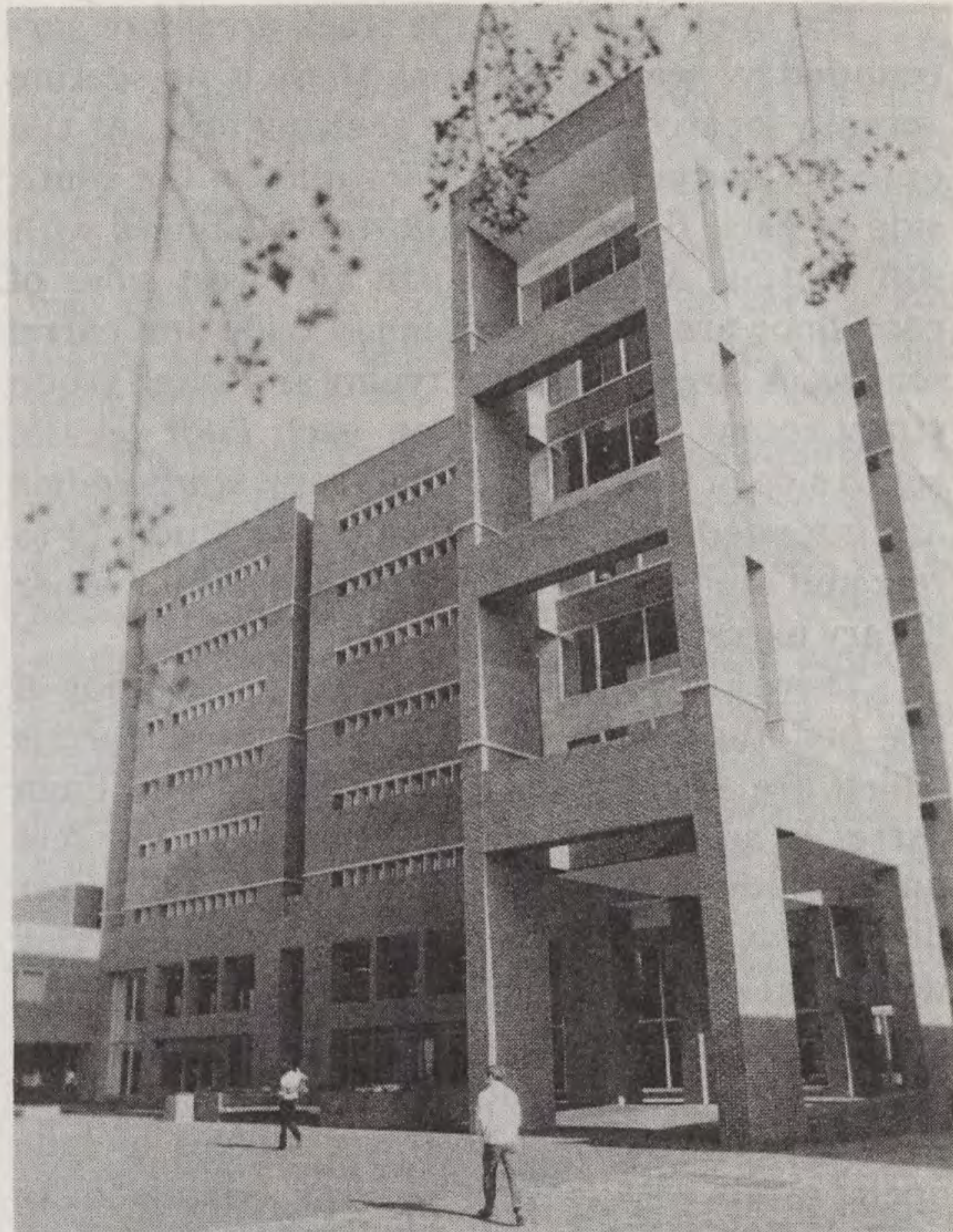
A view of the west end of the Davis Library. The entrance to the building is located at the far left under the arcade. (Photo by Will Owens, UNC News Bureau.)
