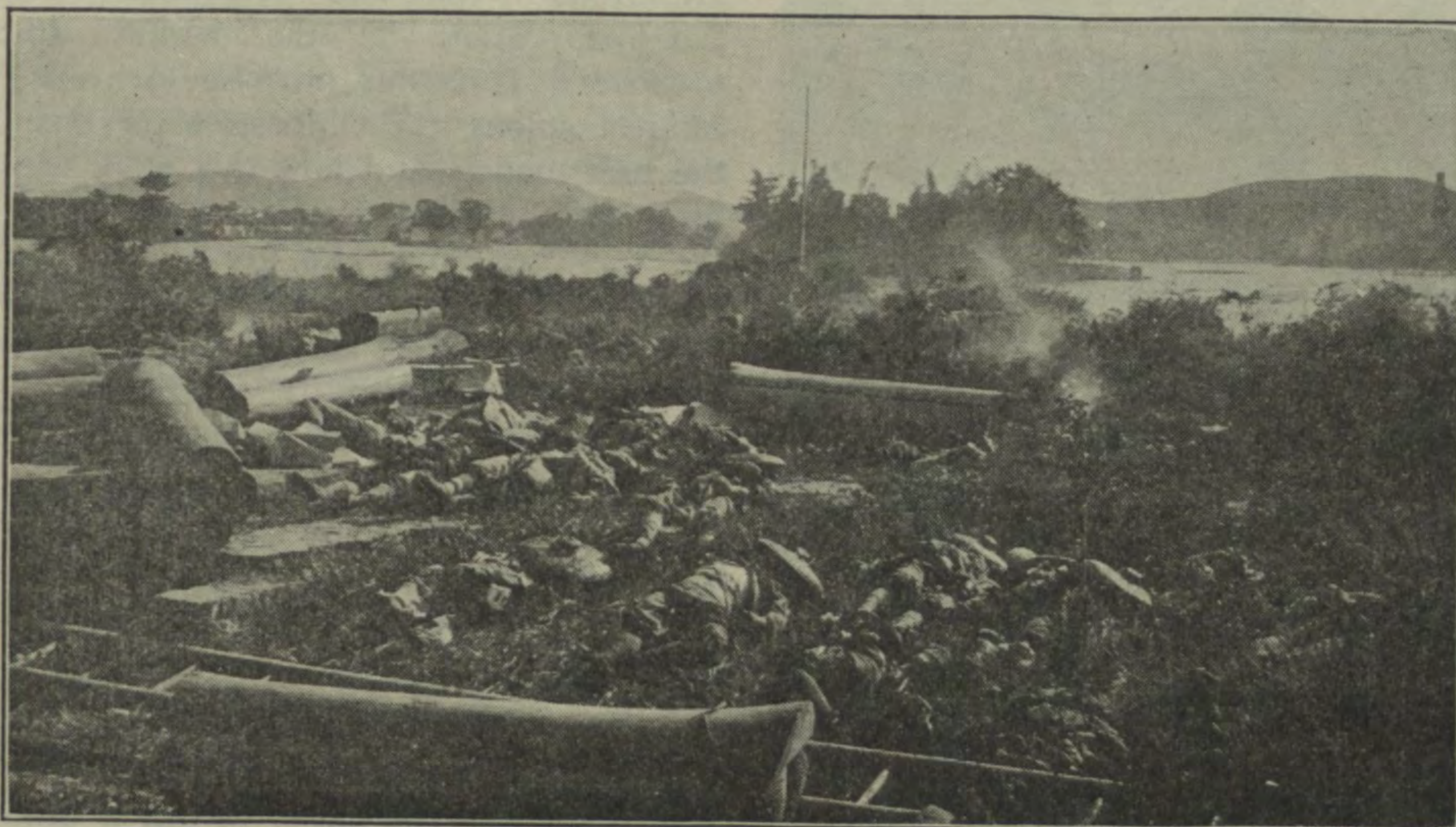
A CROSS OF SUFFERING FOR CHINA
