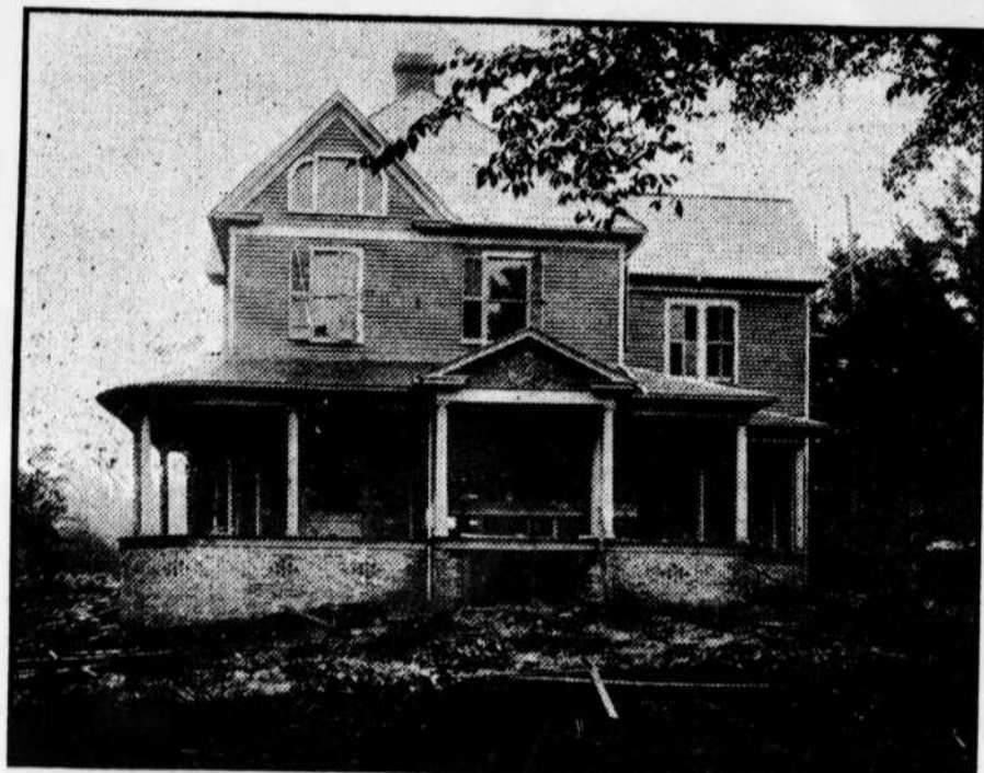
C. S. FORBES' RESIDENCE (under construction).
