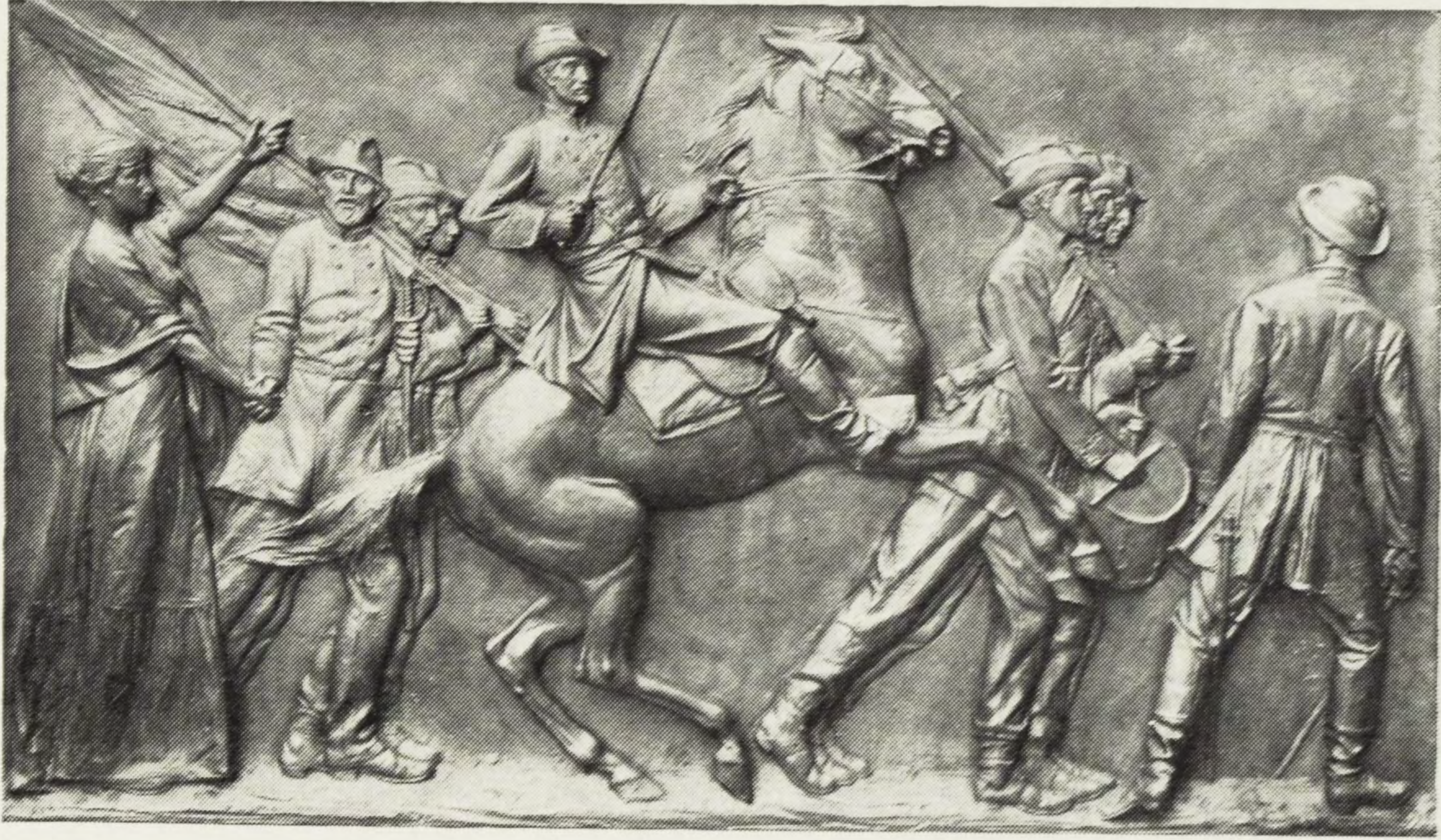
BAS RELIEF ON THE EAST SIDE OF THE PEDESTAL.
