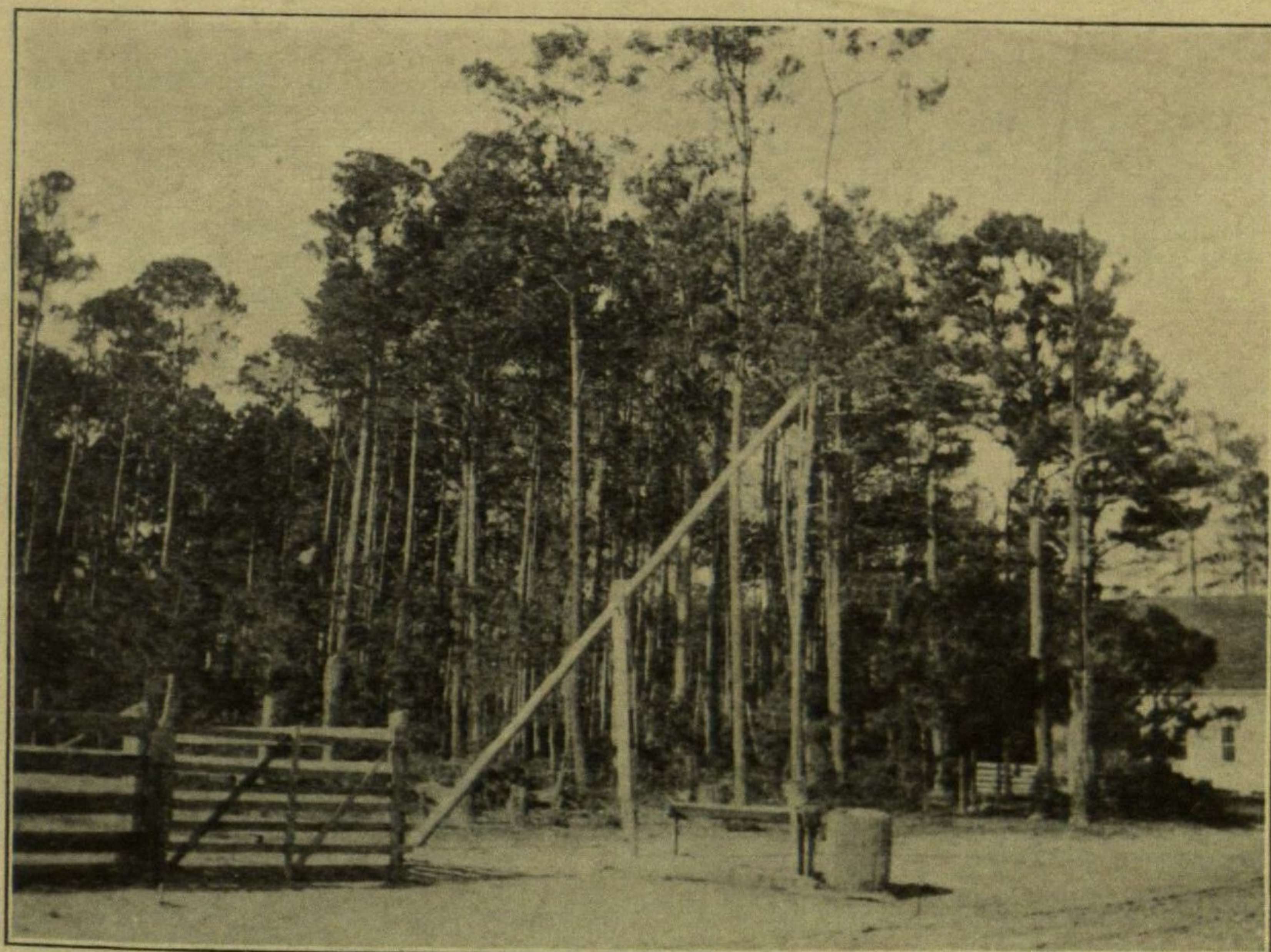
B.—Open well with cypress log curb and sweep lift at Aydlett, Currituck County, N. C.
