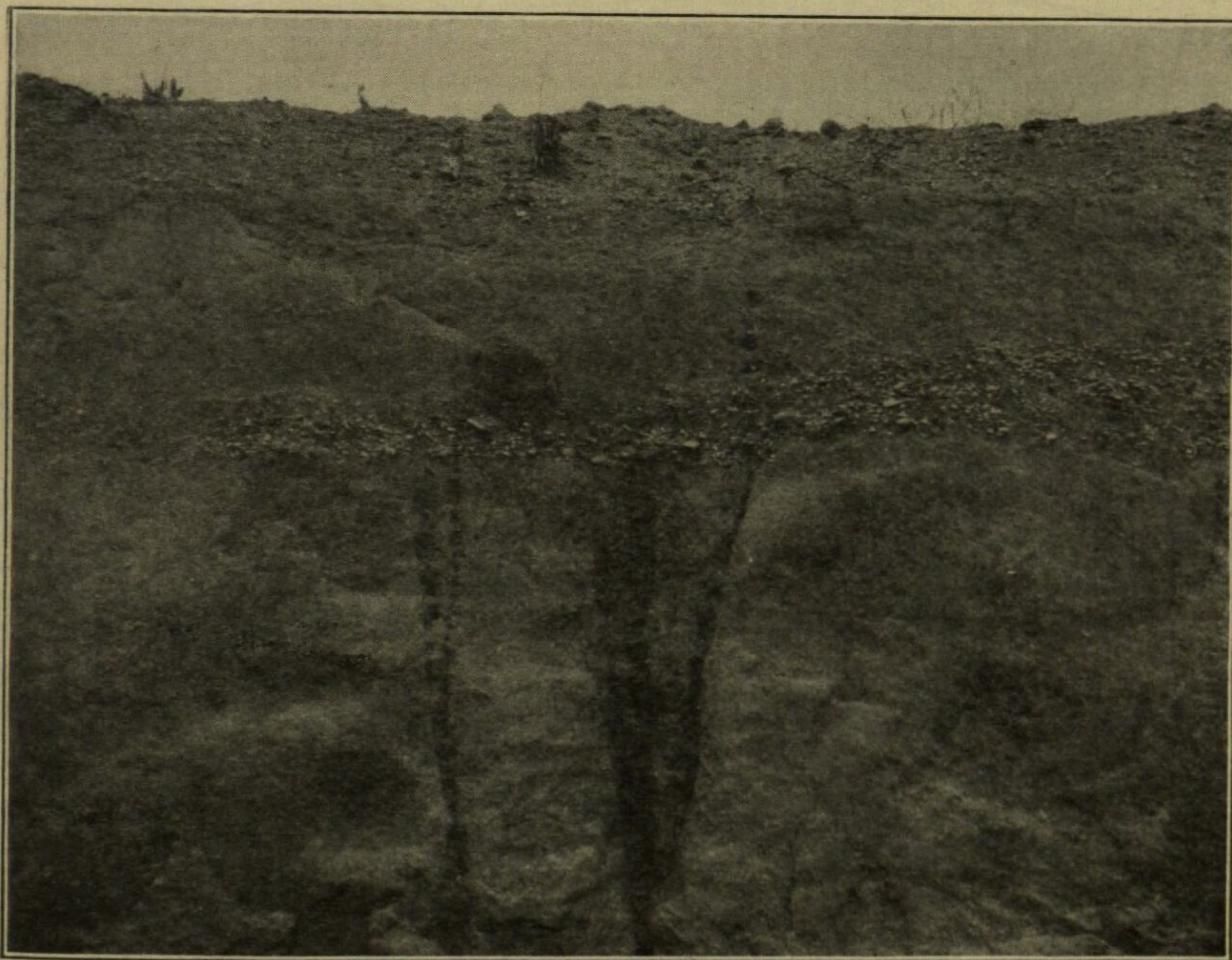
B.—Gravel layer in sand of the Coharie formation; cut of the Atlantic Coast Line Railroad, one mile northeast of Four Oaks, Johnston County, N. C.
