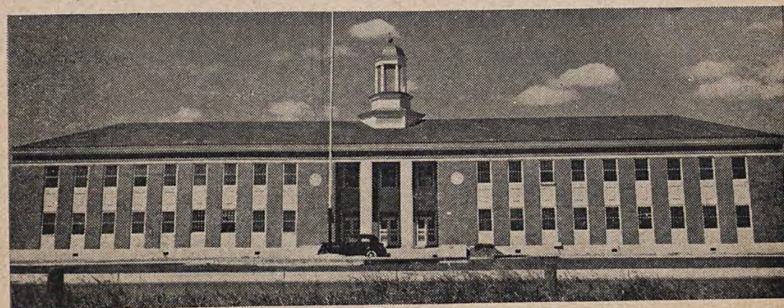
ADMINISTRATION BUILDING IN MAIN AREA AT HADNOT POINT
