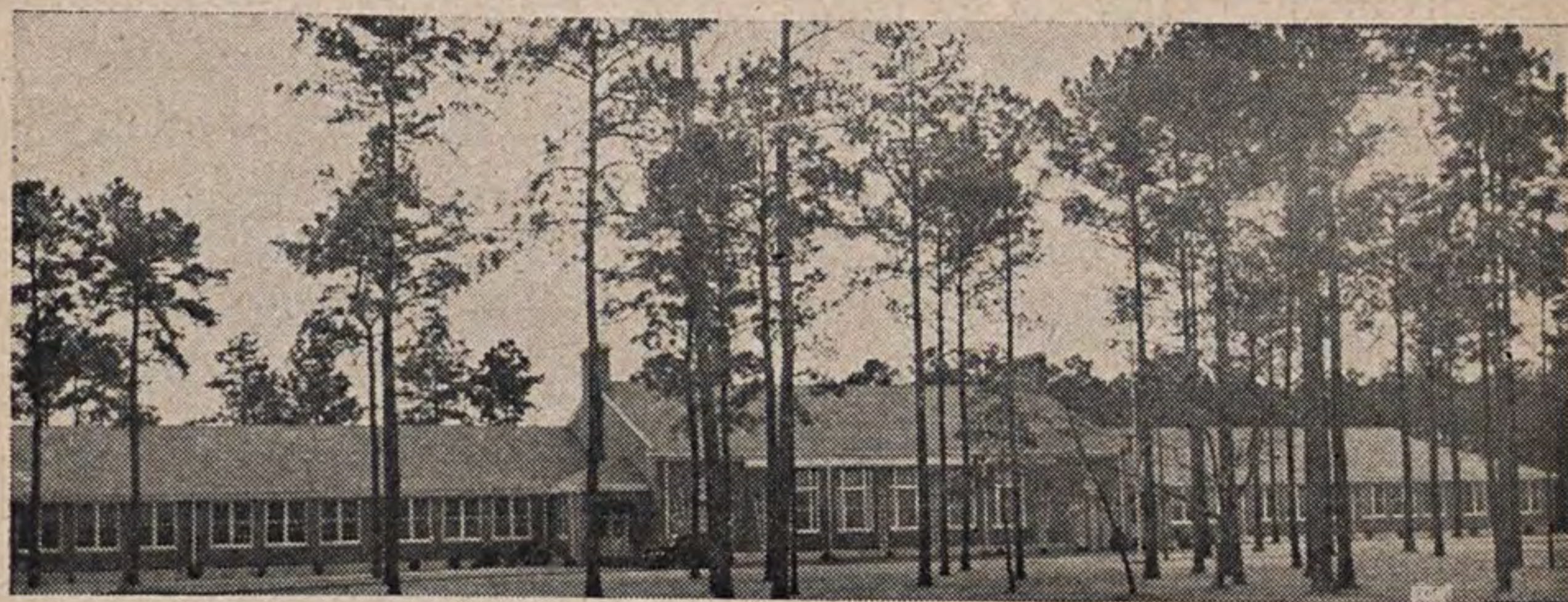
PARADISE POINT SCHOOL LOCATED ON THE RESERVATION
