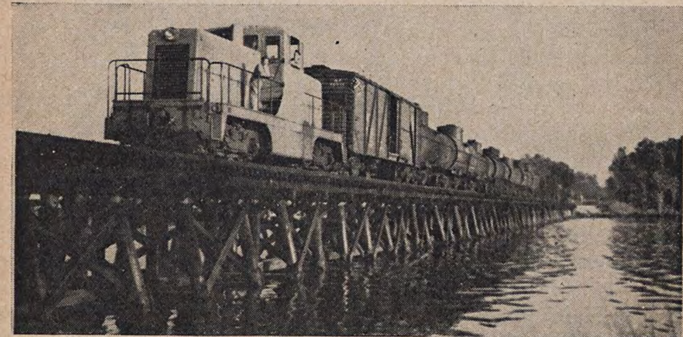
RAILROAD IS PERHAPS THE LONGEST ON ANY MILITARY POST
