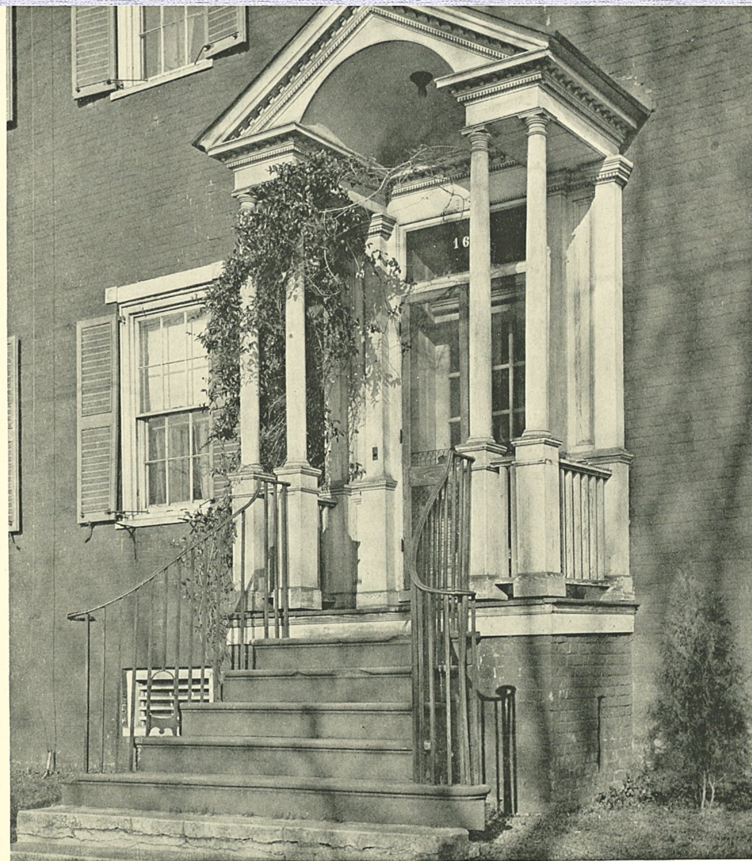
ENTRANCE DETAIL—THE JUDGE DONALD HOUSE, NEW BERN, NORTH CAROLINA
