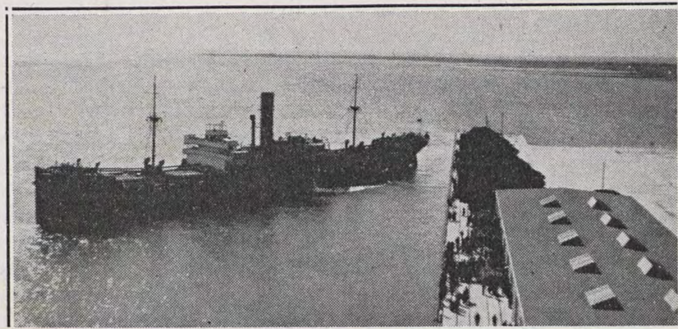
MOREHEAD CITY PORT TERMINAL
