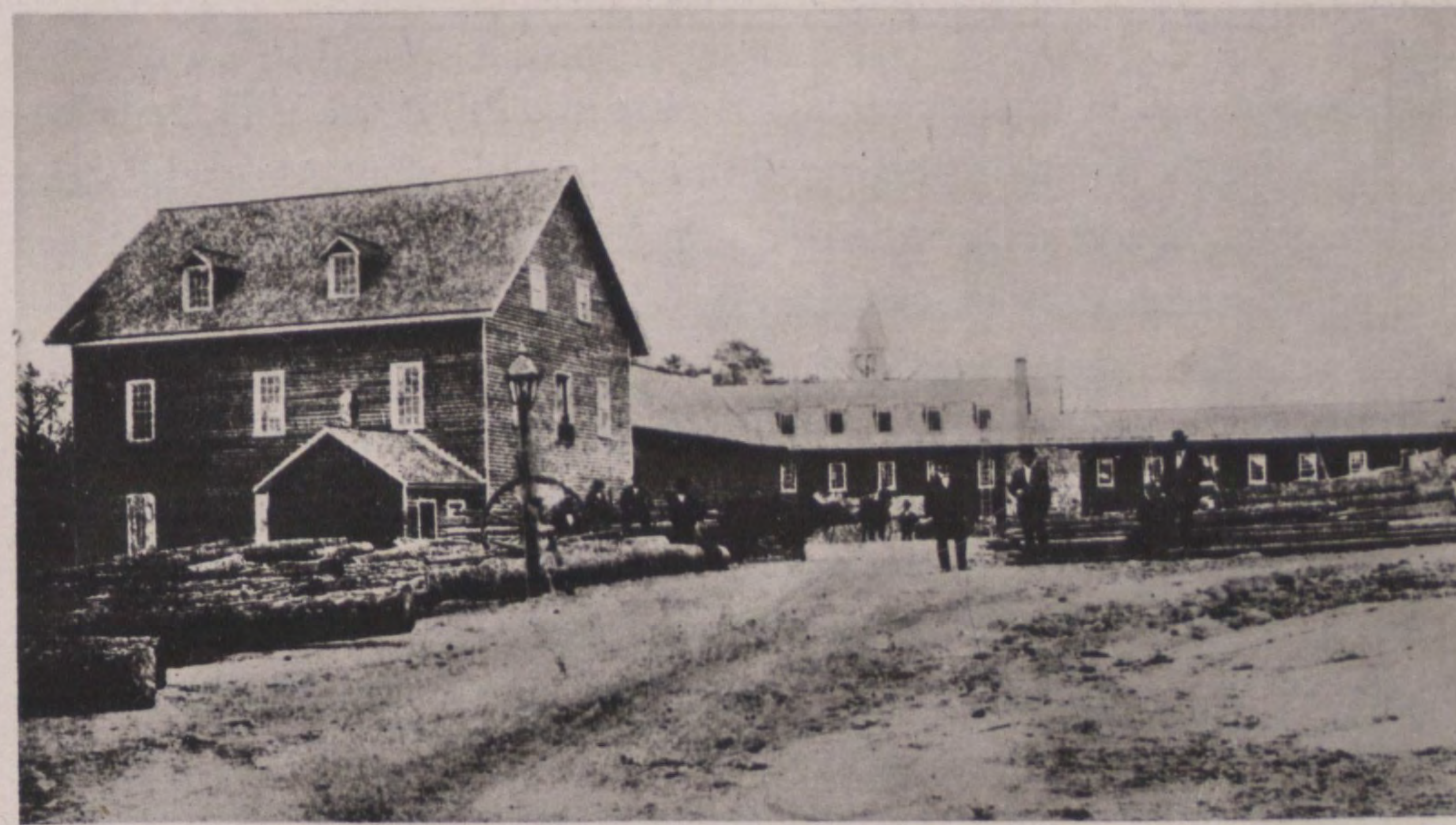
Rocky Mount Mills as rebuilt after the fire of 1869. To the left is the grist mill, then still in operation; to the right, the cotton mill.
