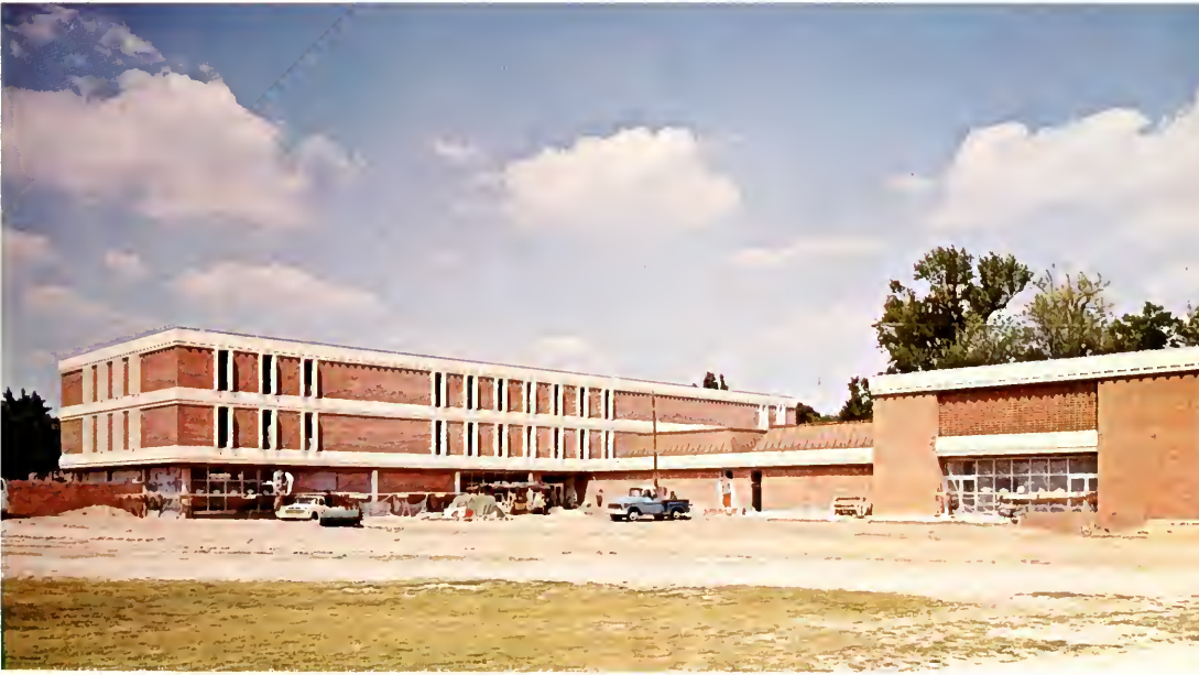
Carpenters and masons add the finishing touches to the new School of Music building
