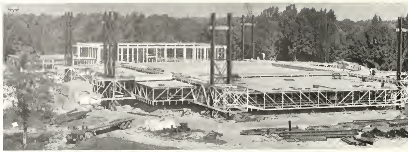
Framework for the roof of Mingus Coliseum is raised, in its entirety, to the top of massive steel pillars.
