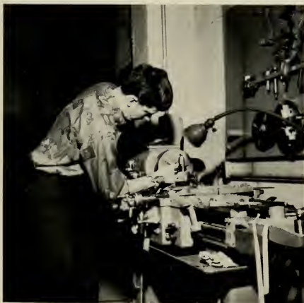
Precision metal tooling can be obtained by a skilled operator of the turret lathe in the Industrial Arts Department.
