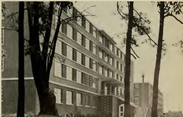
The new dormitories on the south campus house all men students
